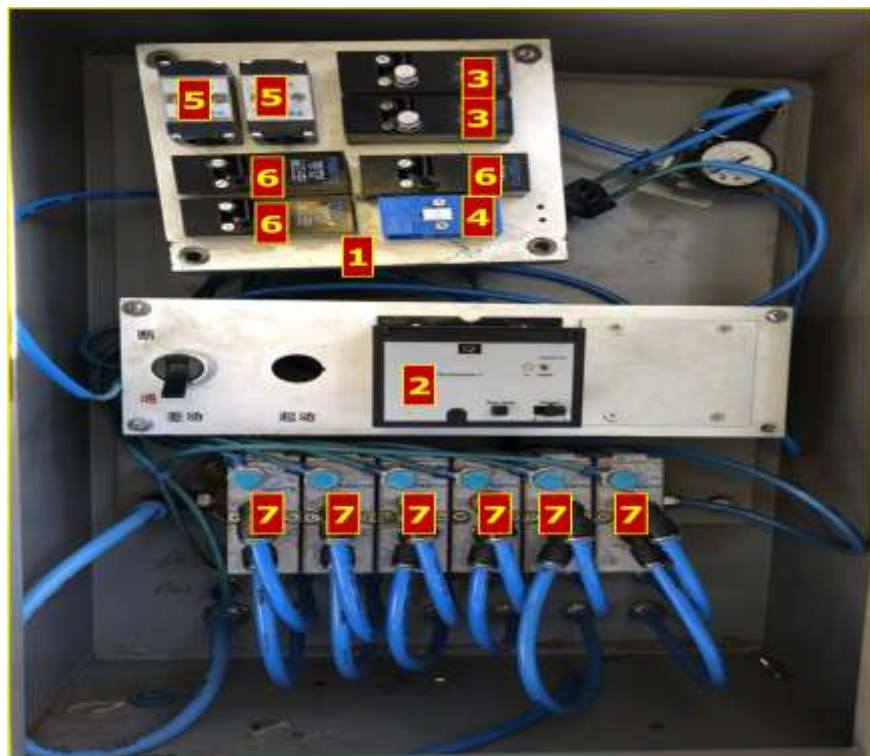
Figure 2-2: Pneumatic Control System Components
