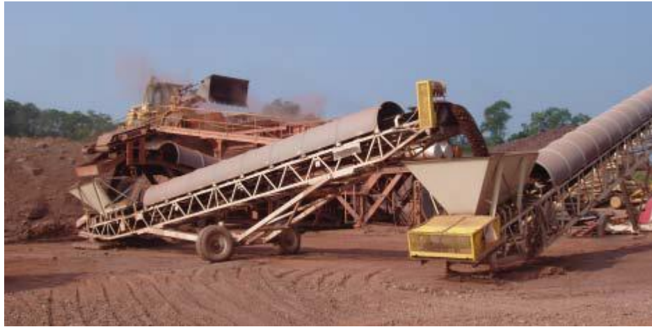
Figure- 3.9 The Clay Crushed and Transported to Storage Area
