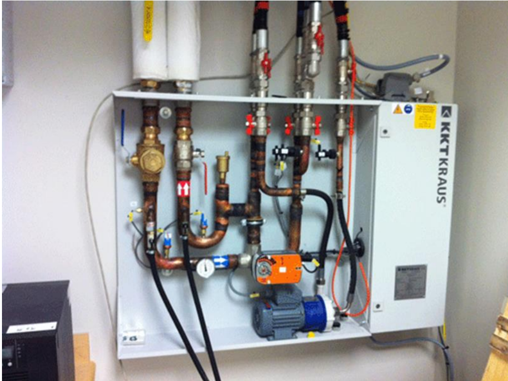
Figure 2.14 Chiller (inside components)
