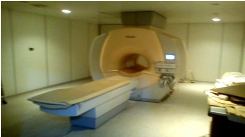
Figure 3.1 Philips MRI machine was used in the study (AlamalDiagnostic Center)
