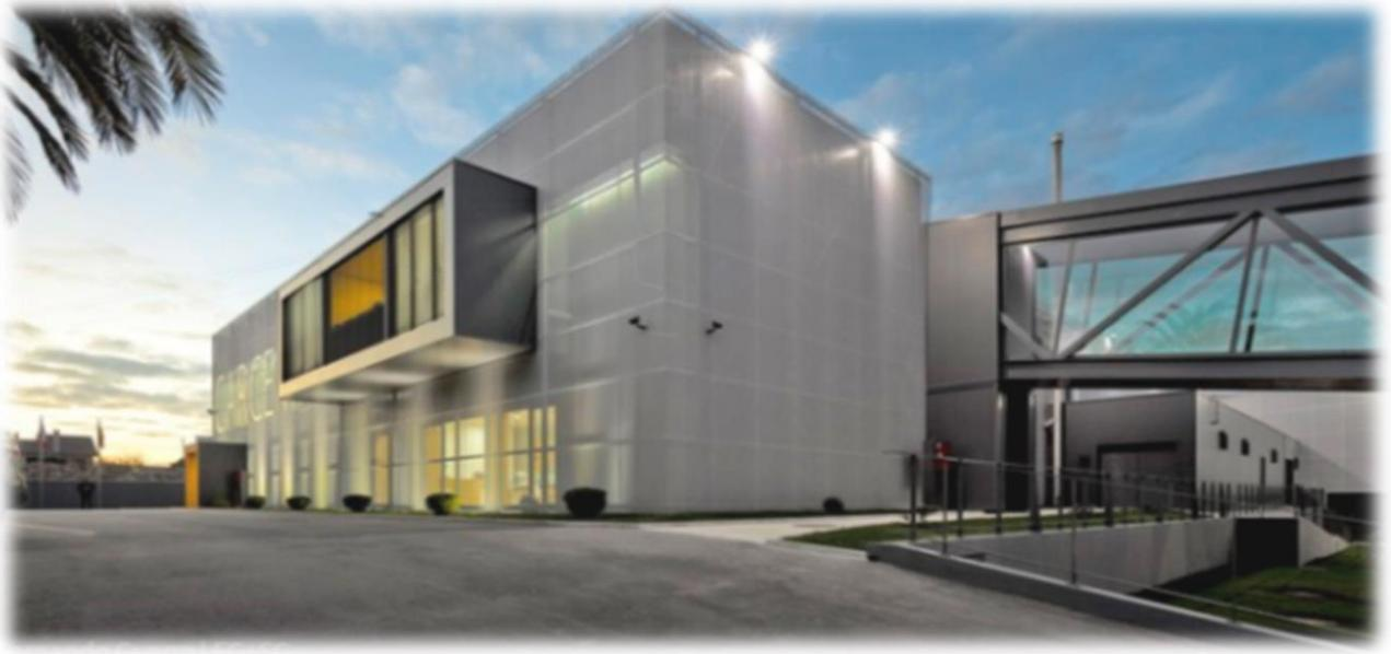
The redesign of the façades and exterior spaces were guided by the concepts of unity and formal homogeneity, leading to an overlay of a new skin in wavy perforated metal sheets along the existing exterior walls. The form, texture and permeability of this skin relates to the fabrics, primary material to the company. This formal analogy is then used in the interior spaces, mainly in the office modules located in the production areas and storage areas.
