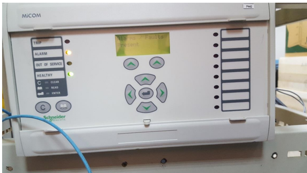
Fig.4.1: MICOM p442 relay.
