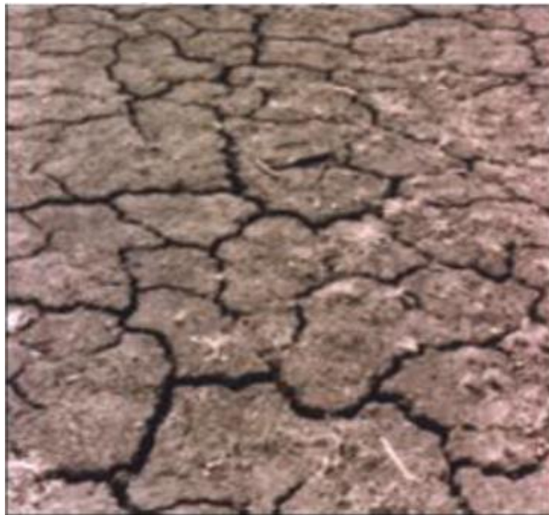
Fig. 3.2 Expansive soil with polygonal patterns cracks
