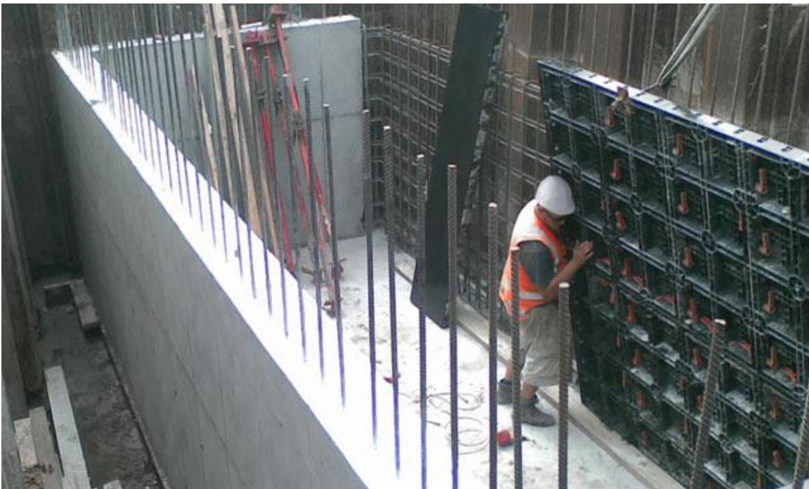
Fig: C.2 Formwork in water tanks
