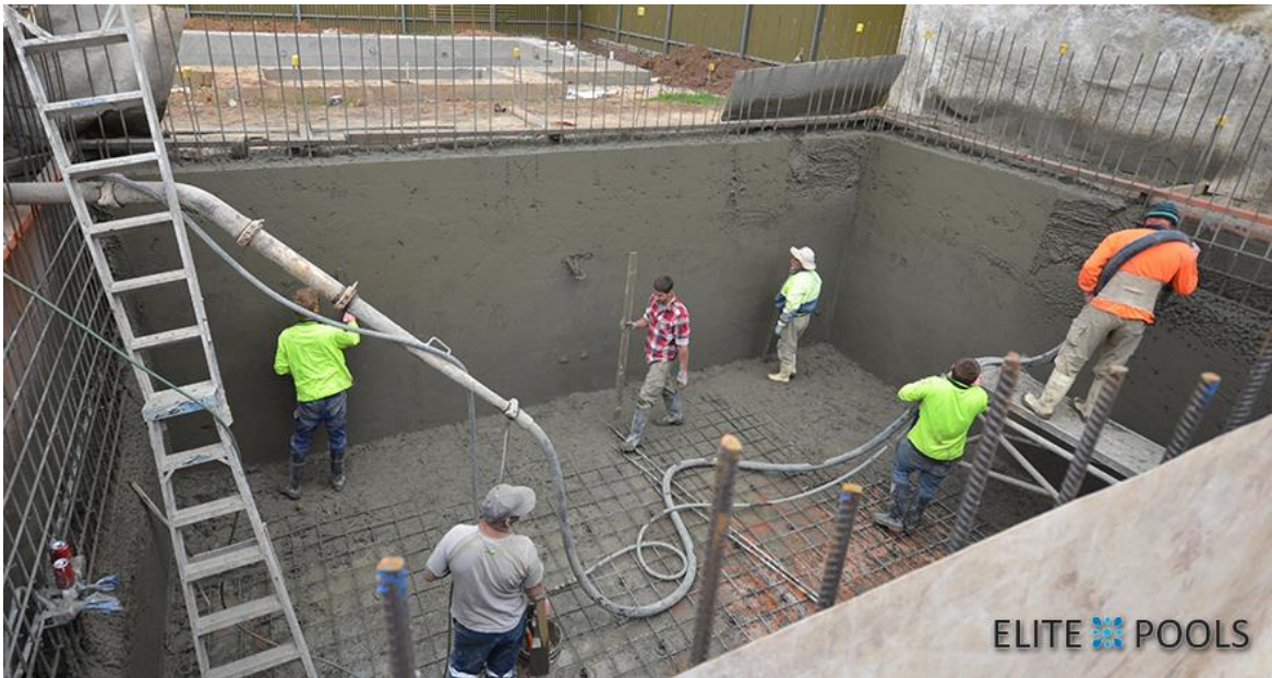
Fig: C.1 Concrete work in water tanks
