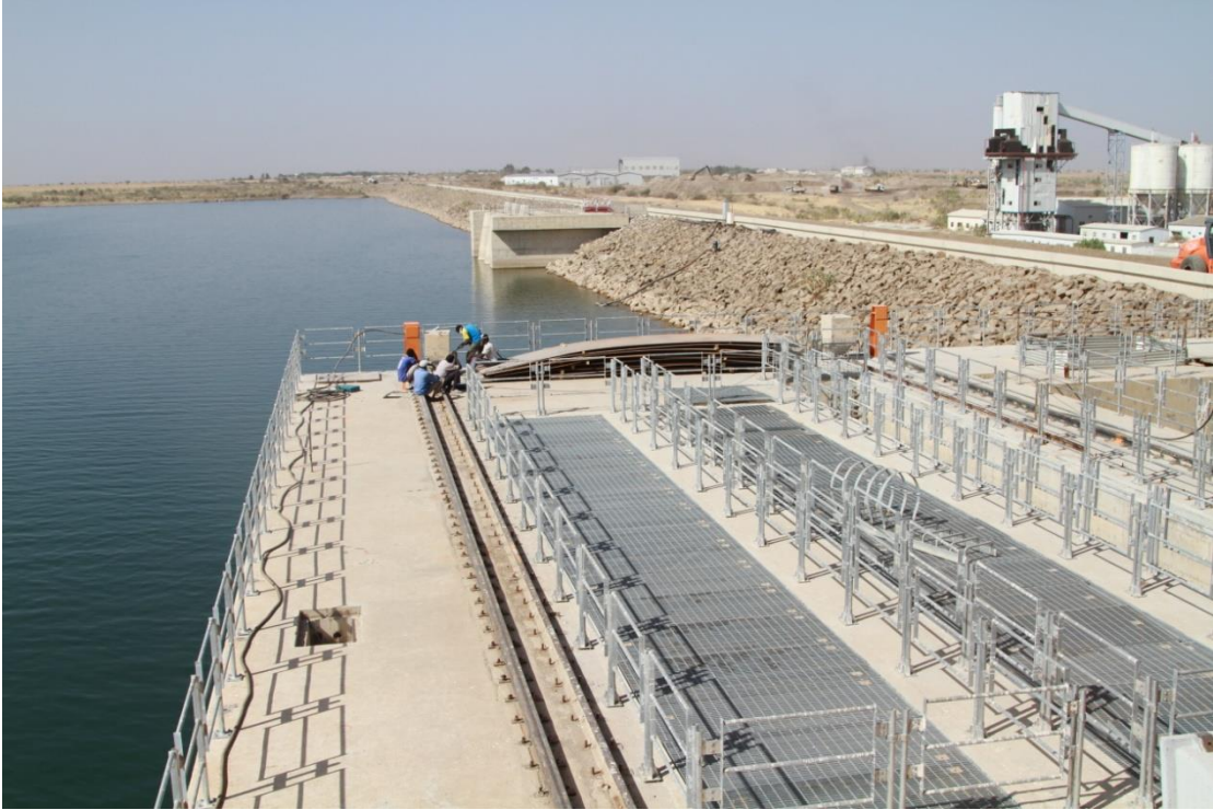
A-7 the Metal Structure
