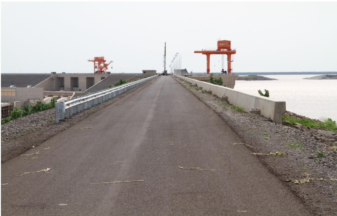
A-9 The Road of Dam Crest
