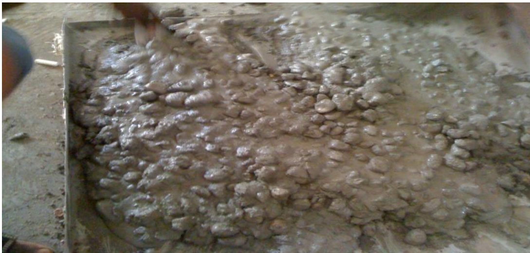
C-2 The concrete mix M (1) with add Superplasticizer admixture
