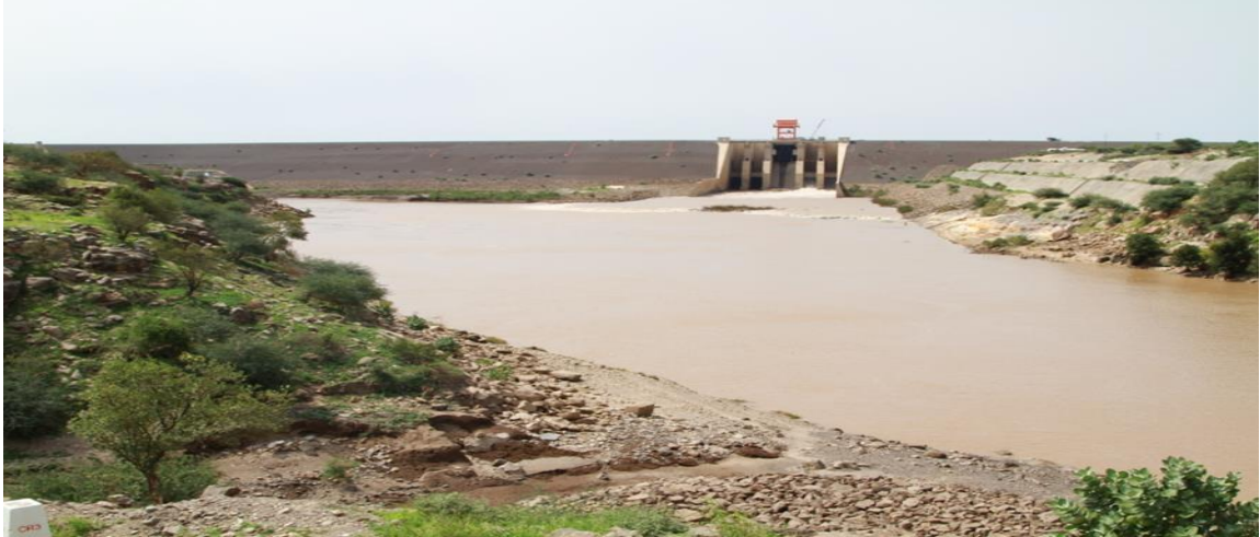
Figure 3-1 General view of The Dam Complex of Upper Atbara Project Downstream
