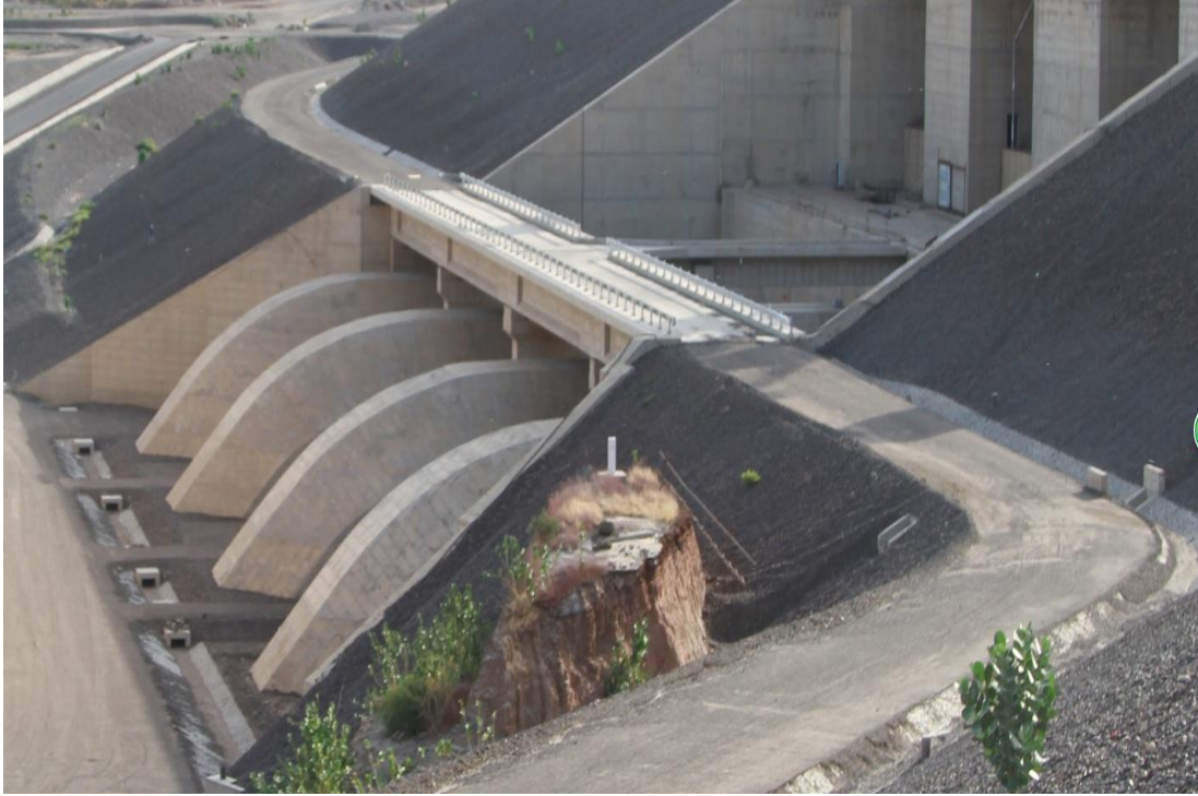
A-3 General View of Traffic Bridge
