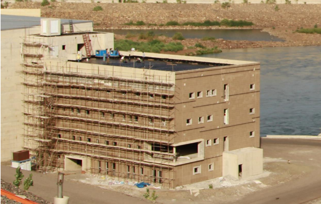
A-5 General View of Operation Building
