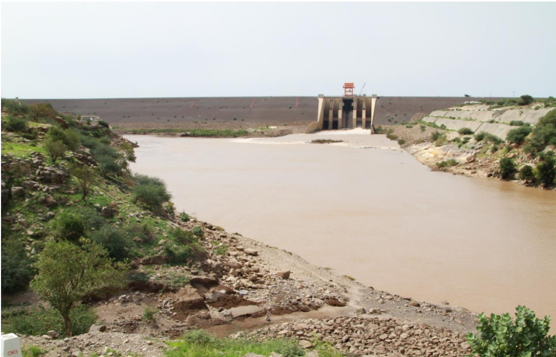
A-2 General view of Downstream
