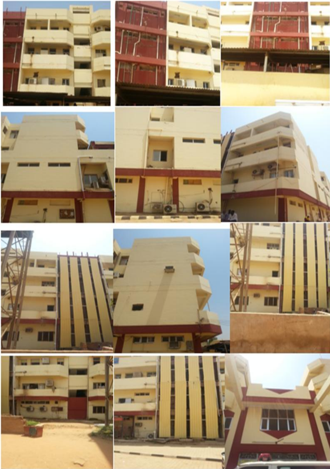
Fig 5.2 Several Photos “scanning” the departure the Emergency (outside)
