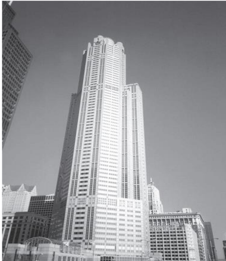
Figure 2-2: South Wacker Drive, Chicago – high strength concrete used in columns.
