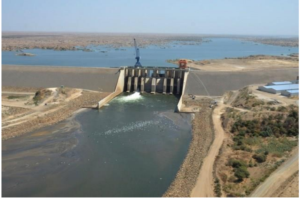
Figure 3-3: Upper Atbara Spillway
