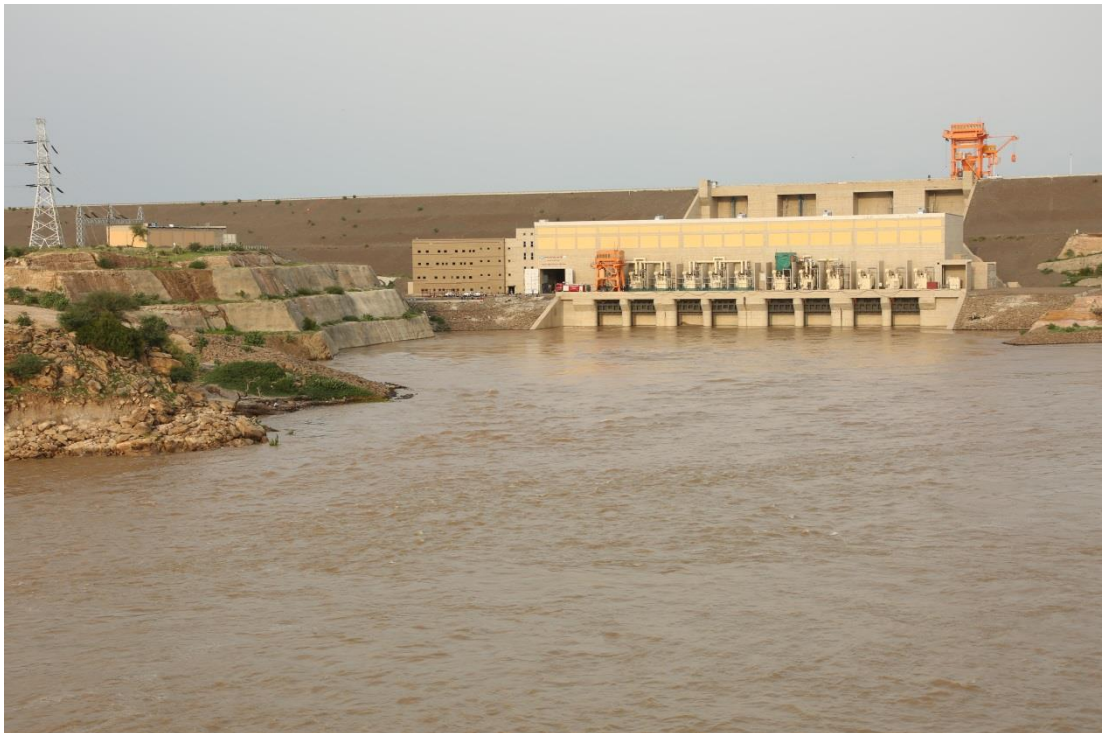
Figure 3.2: The Power House
