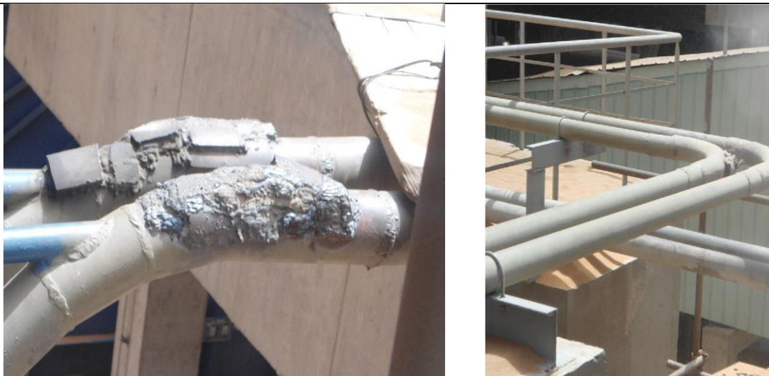
3- Failure in elbows
