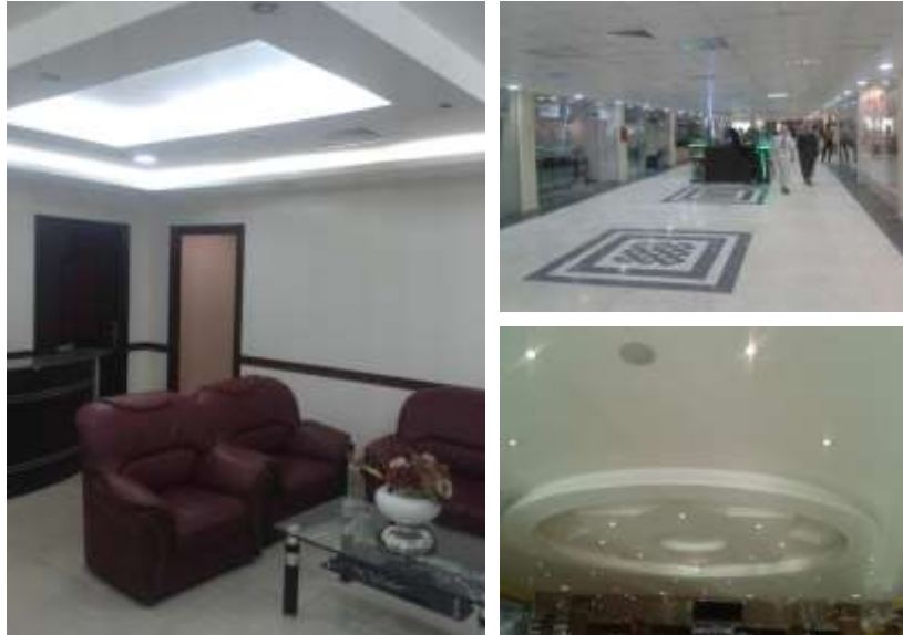
Figure (4-17) gypsum boards (dry wall) and aluminum suspended ceiling (Afraa mall) Source (the researcher)
