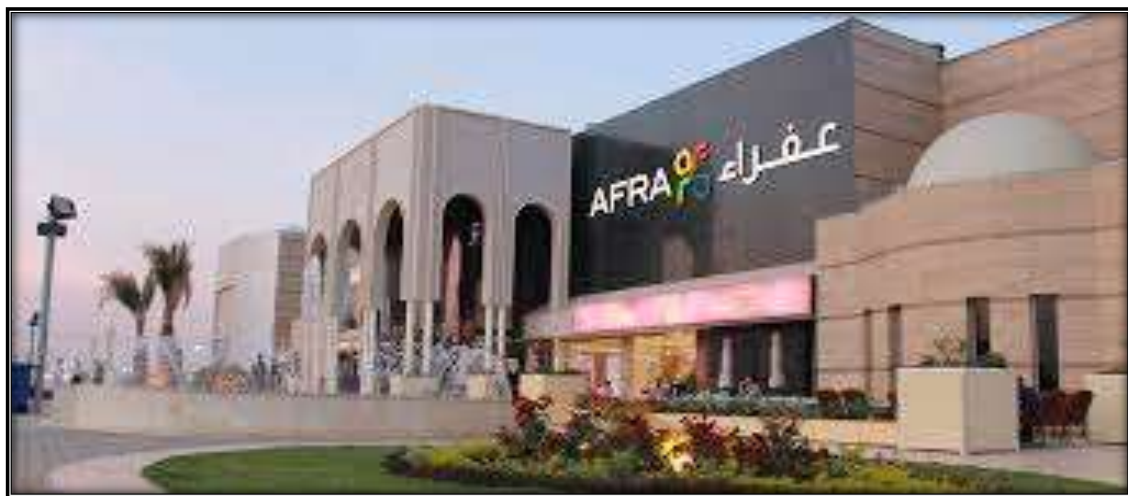
Figure (4-8 ) Afraa mall project – Main Entrance
