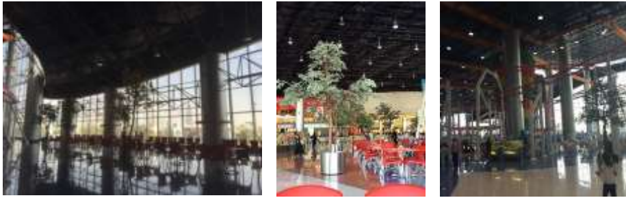
Figure (3- 29) Appearance of the structural elements inside the space
