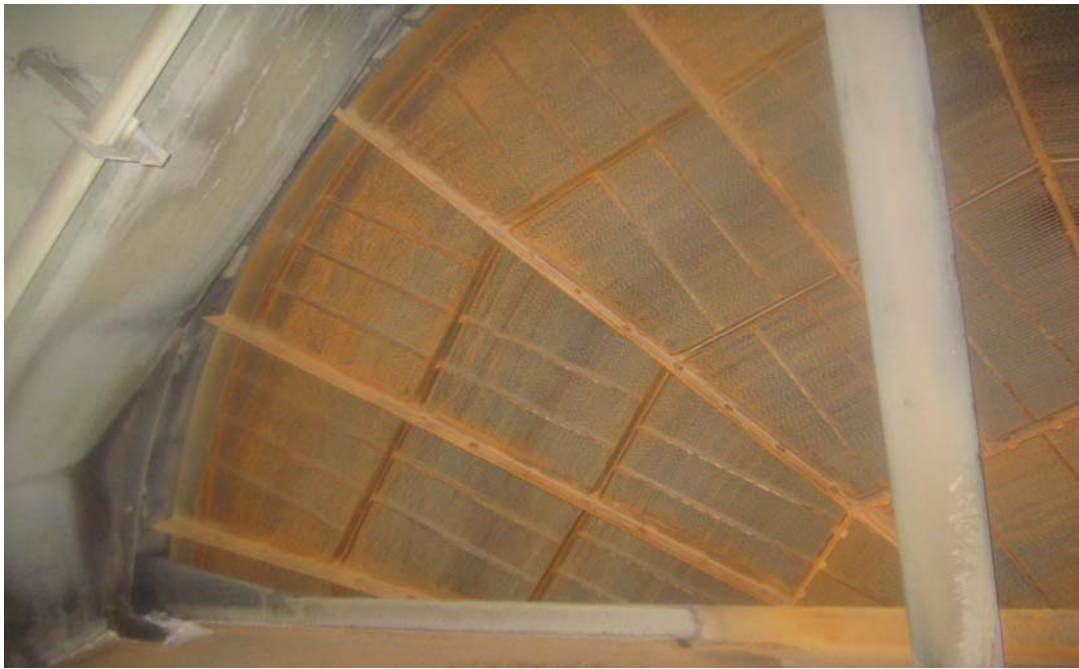
Figure 2.14: Internal side of Rotary Air heater.
