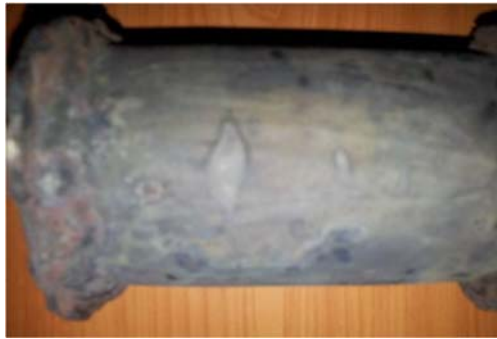
Figure 2.20: Failure caused by Corrosion fatigue.
