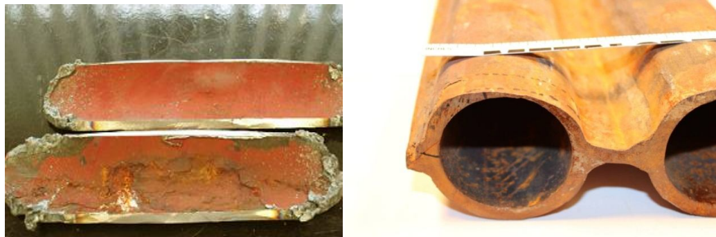
Figure 2.22: Failure caused by internal erosion.
