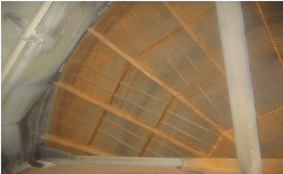
Figure 2.14: Internal side of Rotary Air heater.
