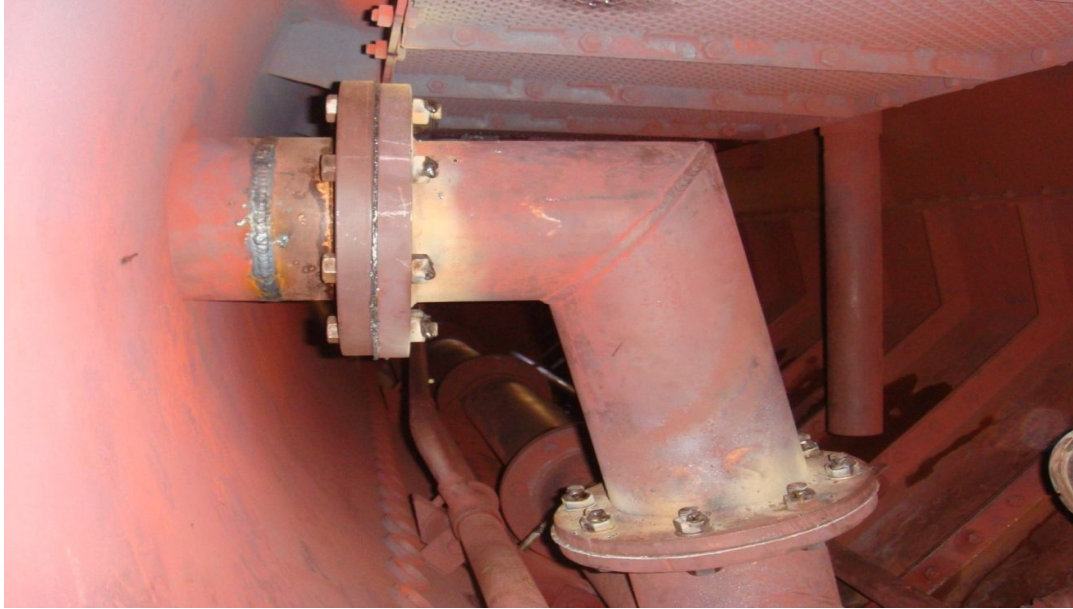
Figure 2.12: Internal side of boiler drum.
