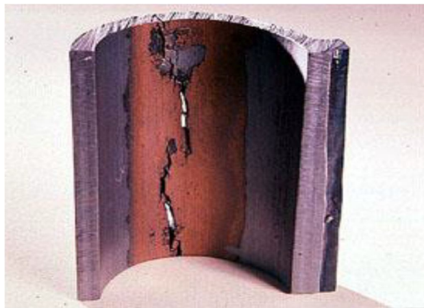
Figure 2.23: Failure caused by internal corrosion
