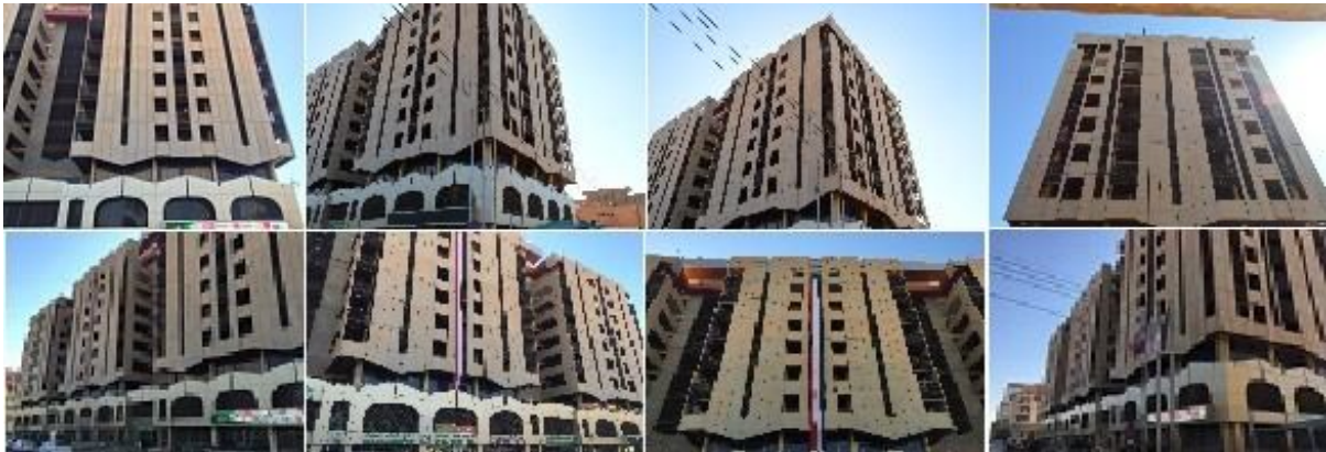
Figure 5.3: Several Photos “scanning” of building (the front)
