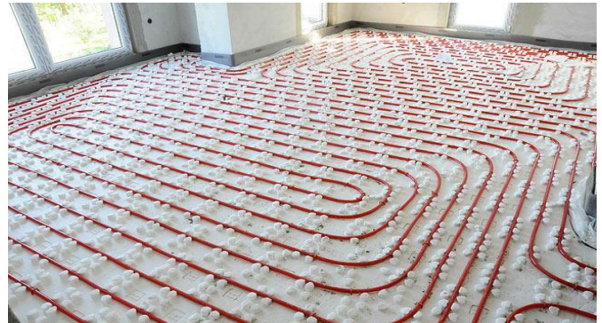
Figure 5-25: Hydronic Radiant Floor Cooling
