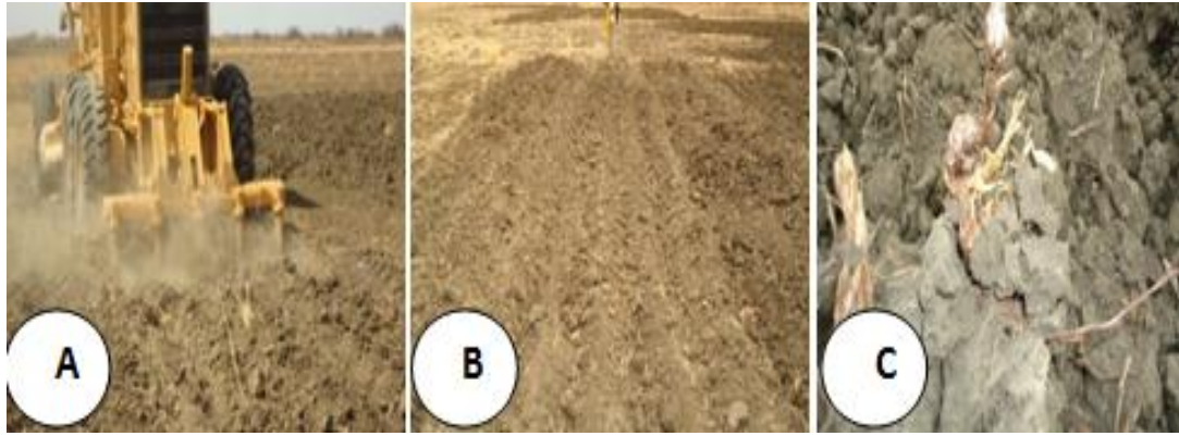
Appendix 3. Modified machine. A) in action, B) soil surface after blading and C) tubers in a clod
