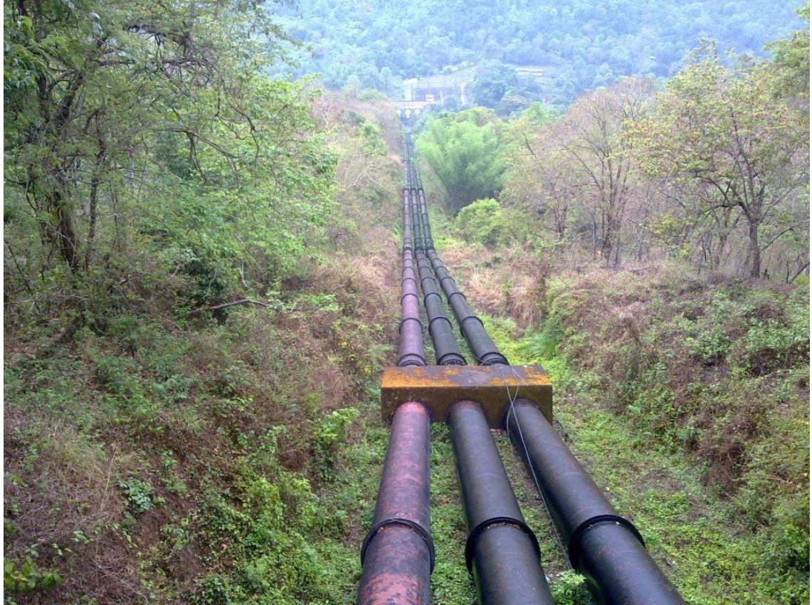
Figure (3.3) Shape of Penstock.
