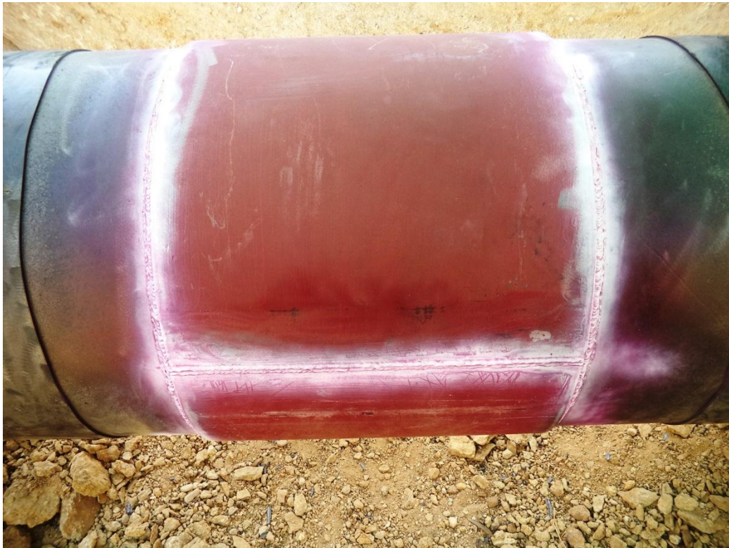
Fig. (6. 8) Illustration of a Type B sleeve
