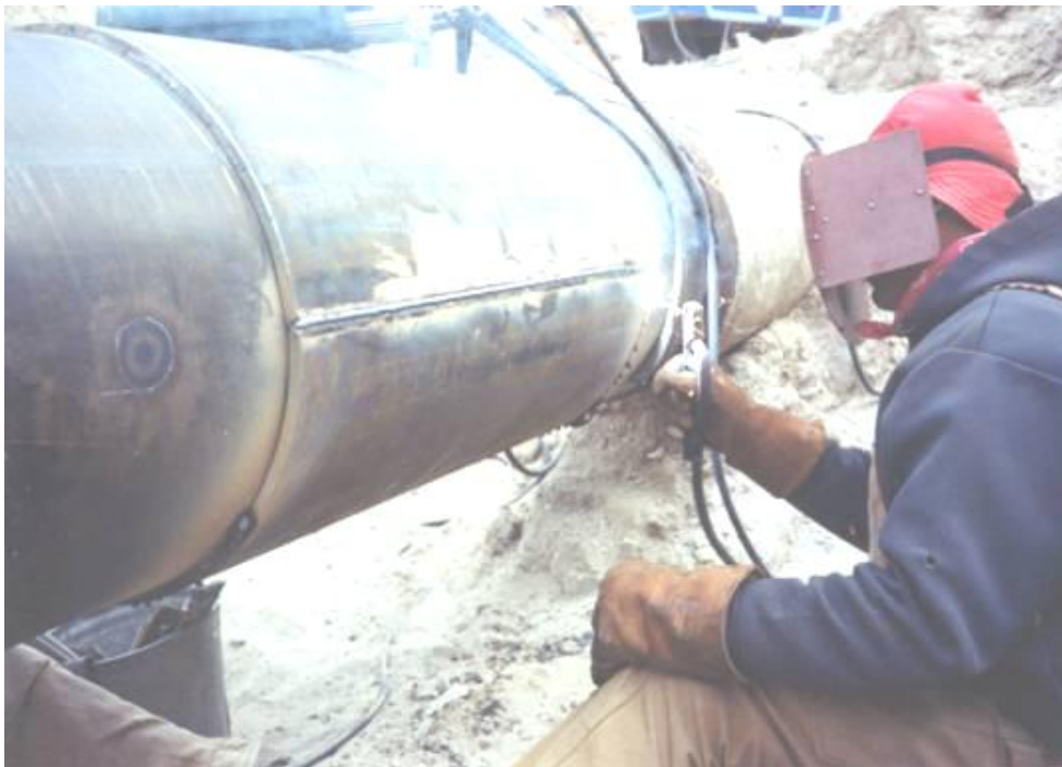
Fig. (6. 7) Installation of a Type B repair sleeve
