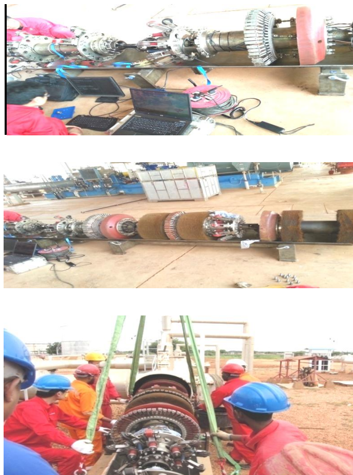
Fig. (2. 2) IP Inspection for HC Pipeline
