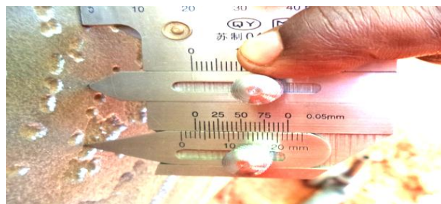
Fig. (2. 1) inspection Pipe Corrosion
