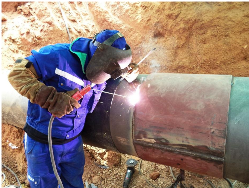
Fig. (6. 2) Weld details for Type A sleeve
