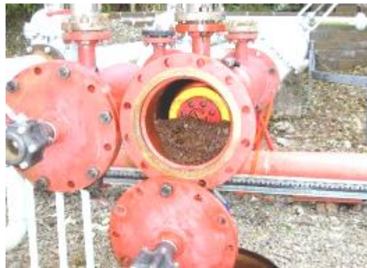
Fig. (3. 1) Debris after pigging
