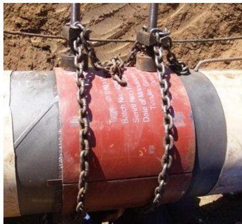
Fig. (6. 3) a Lug and Bolt Method
