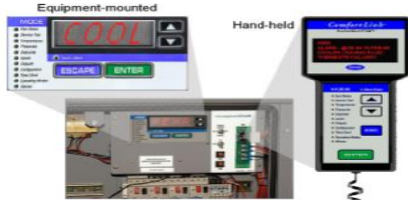
Figure (2.6):Chiller control
