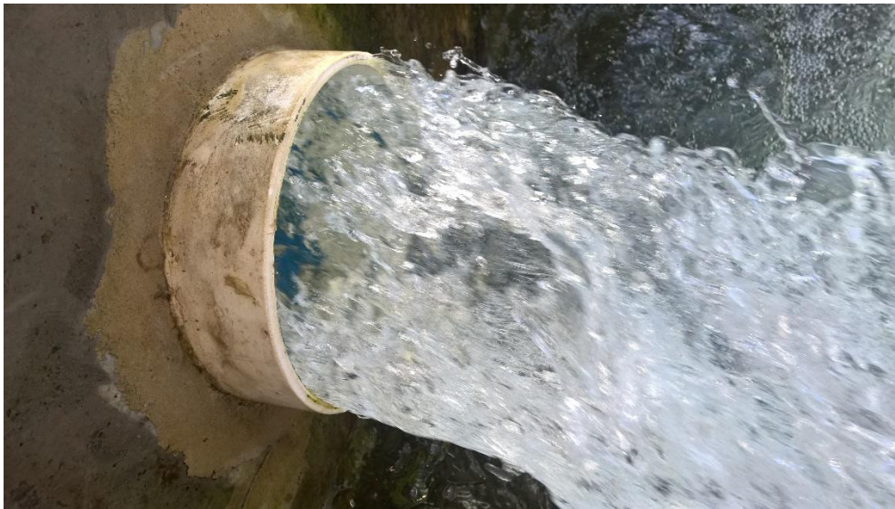
Figure 4-15 : Clear water of seepage pipe.
