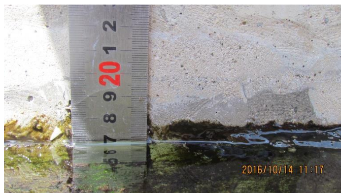
Figure 3-13 : Measurement of water head at seepage weirs.
