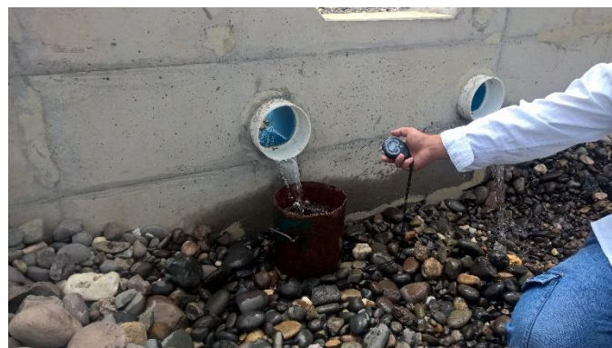
Figure 3-12 : Measurement of seepage pipes.
