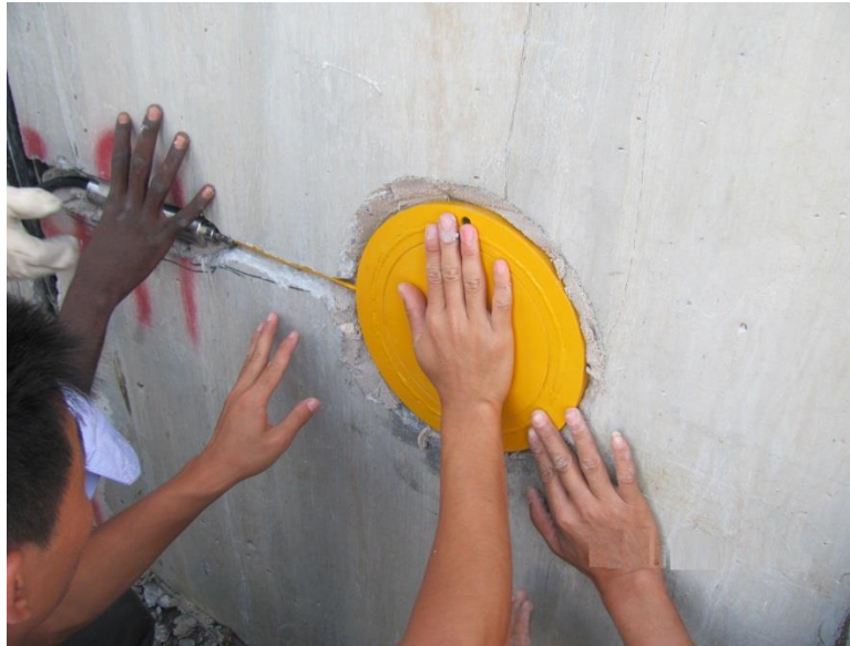
Figure 3-10 Fixation of pressure cells in the concrete face.
