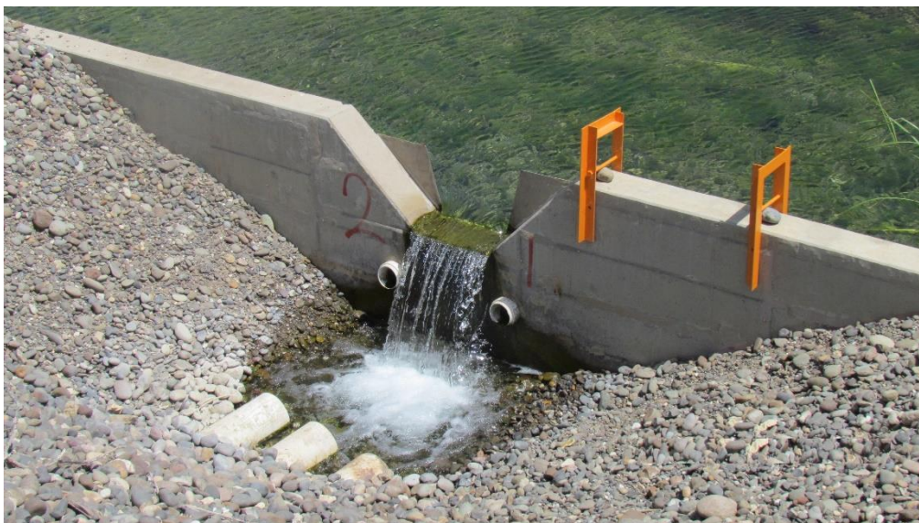
Figure 4-16 : Clear water of seepage weir.
