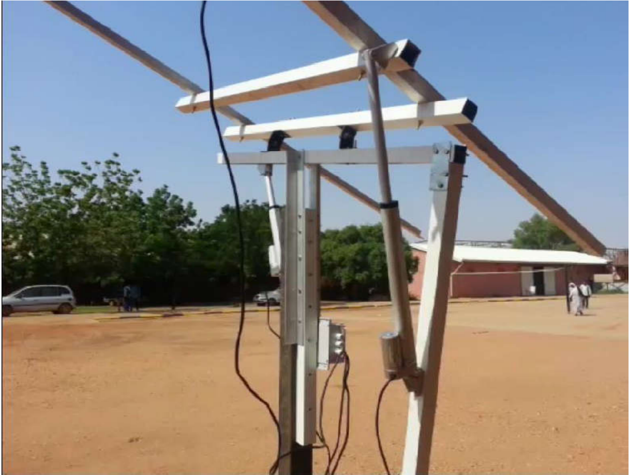
Figure 4.2: The final structure of tracking system
