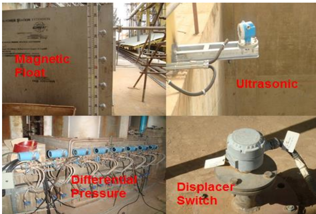
Figure (2-9) different level sensors for boiler
