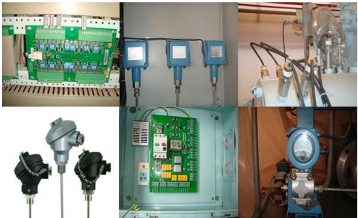
Figure (2-8) sensors installing on the boiler
