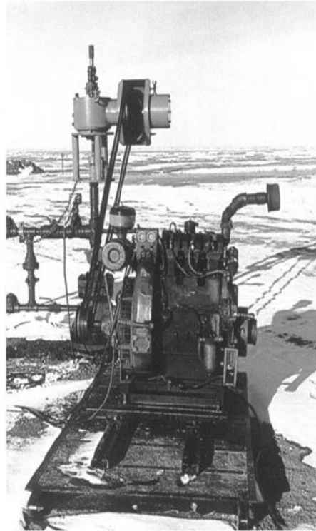
(b) Gas engine direct drive system.
