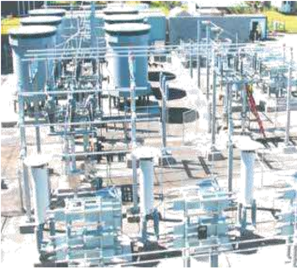
Figure A. 5 Directly connected SVC
