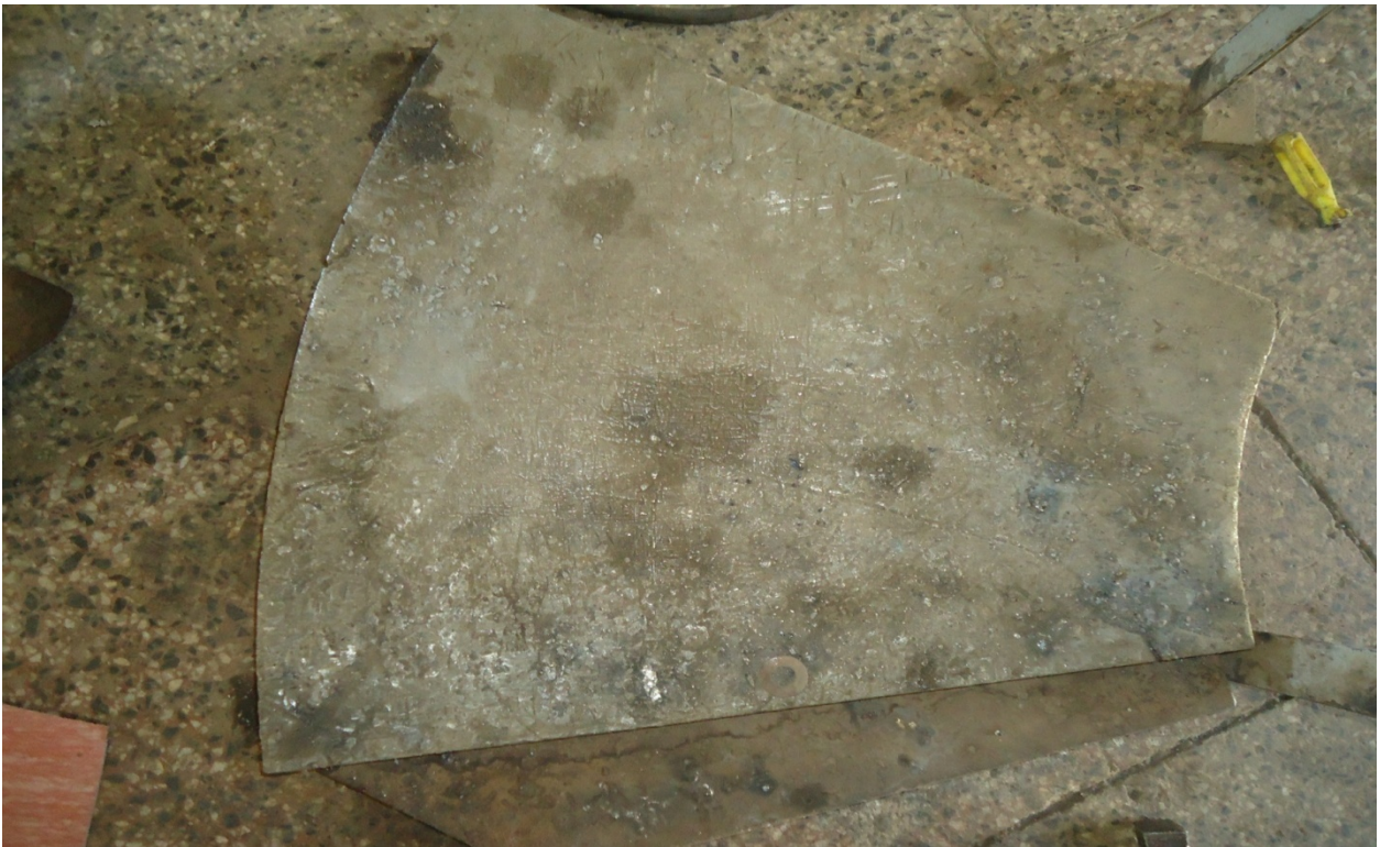
Figure (2.11) Turbine Guide Bearing
