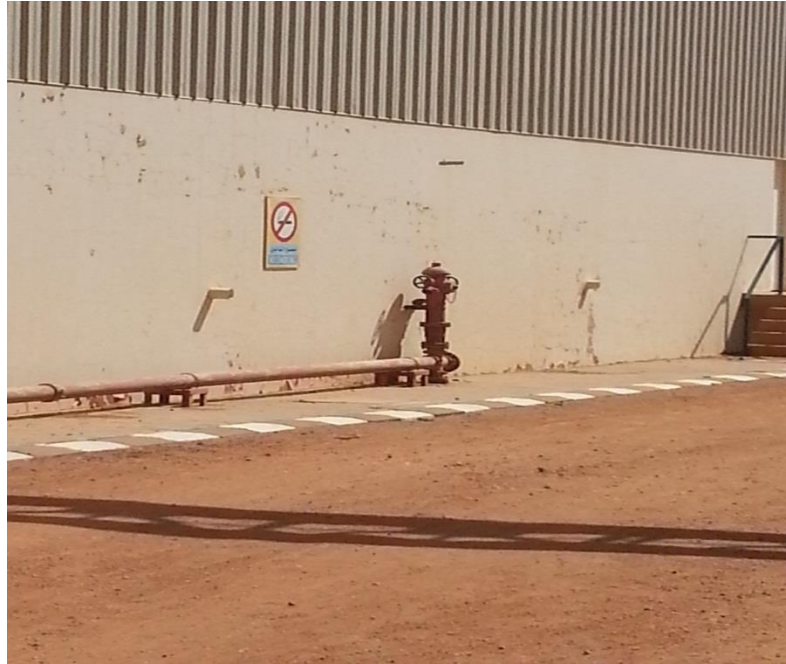
Figure 2.2: Fire Hydrant.
