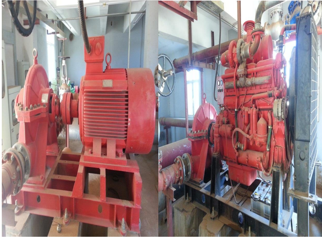
Figure 2.1: Firefighting Pumps.
