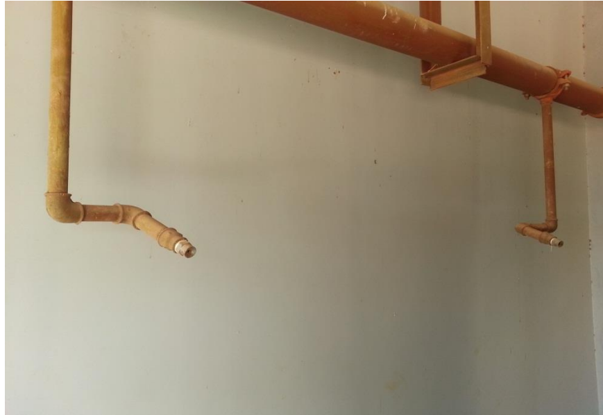
Figure 2.3: Sprinklers
