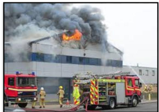
The Figure (2-6) shows fire in factory http://www.safety4arab.com , 2016.
