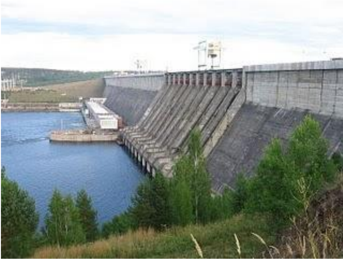
Fig No (2.7) Concrete Gravity Dam North of Irkutsk, Russian Federation ( www.hydroelecricc.energy.blogspot.com )
