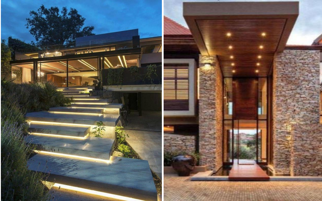
Figure (2-8) the introductory space for residential building
