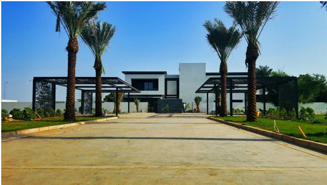
The figure (4-24) main entrance
