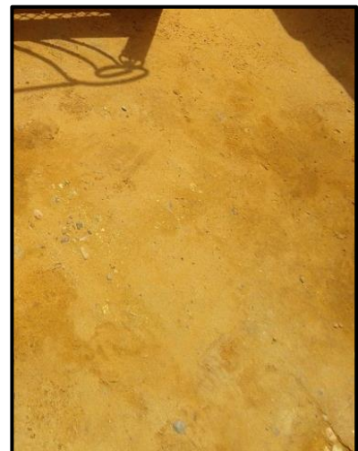
Front yard floor which finished with loose Sand
