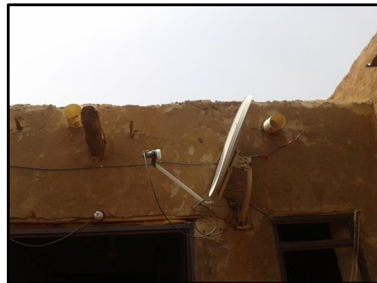
External walls finishing using plaster and a layer of white lime wash
