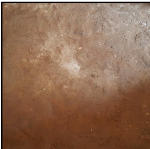
Hall's floor which is finished with Mud mixed with gravel
