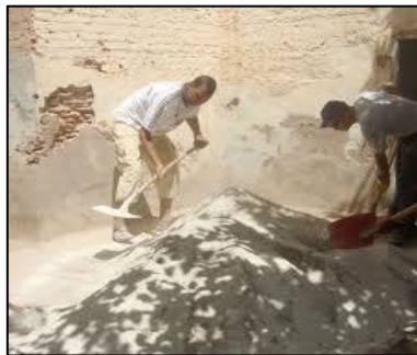
White lime mixing with mud
