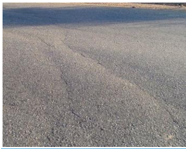
Fig. A.10: Low Severity Upheavals and Settlements
