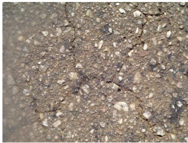
Fig. A.7: Low Severity Block Cracking
