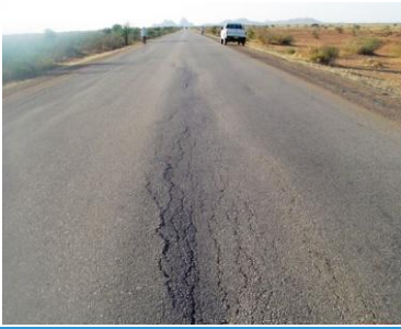
Figure A.42 Medium Severity Rutting
