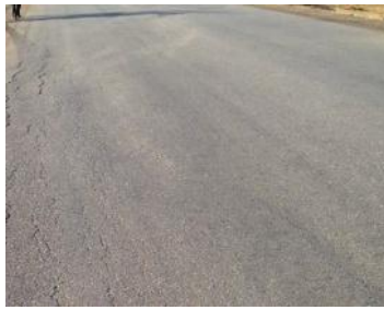
Fig. A.10: Low Severity Upheavals and Settlements
