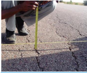
Fig. A.17: Medium Severity Depression
