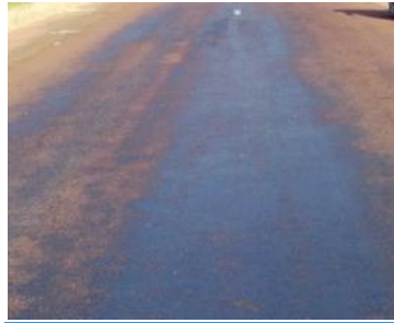
Fig. A.4: Low Severity Bleeding
