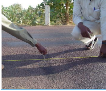
Fig. A.16: Low Severity Depression
