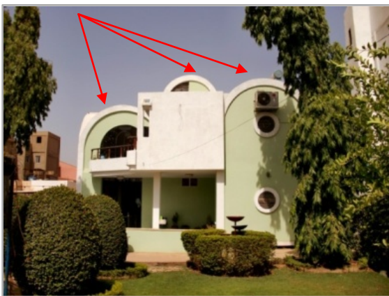
Fig.4.57 Vaults used in the house.
