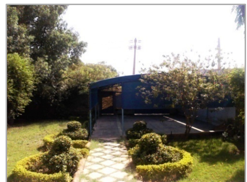
Fig 4.30 Main entrance gate with landscape.
