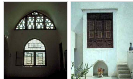
Fig 3.36 In and out view of the wooded window Source: Hassan Fathy/editor, Ismail Serageldin, 2007).
