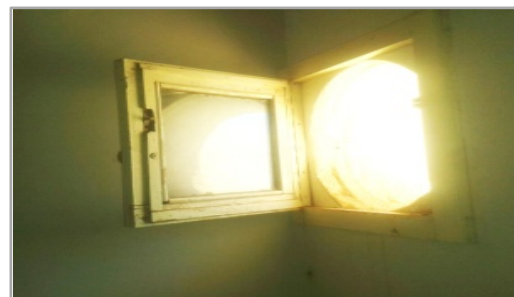
Fig.4.45 Ventilation window in mezzanine floor
