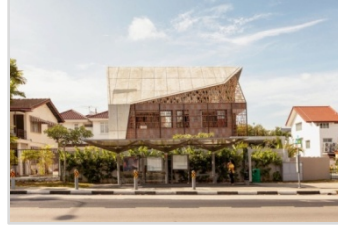
Fig.3.26 Main elevation of the house. Source: https://www.archdaily.com/789395 , 2016.
