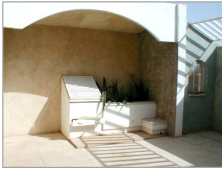
Fig.4.49 Wind catcher with plant beds (Before and after execution).
