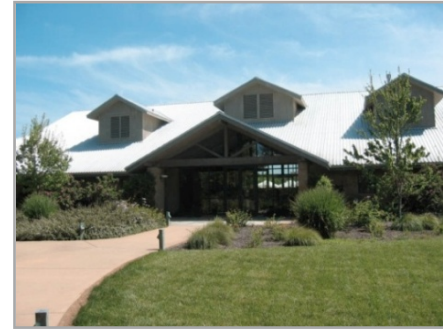
Fig.2.31 Fetzer winey administration building entrance.
