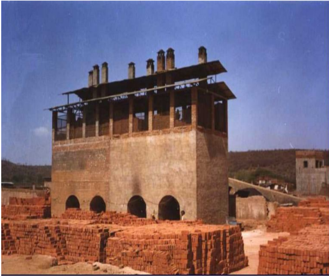
(B-7) Multi- Vertical Shaft Brick Kilns
