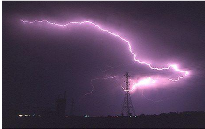
Fig 2.4- Lightning strike – transmission tower
