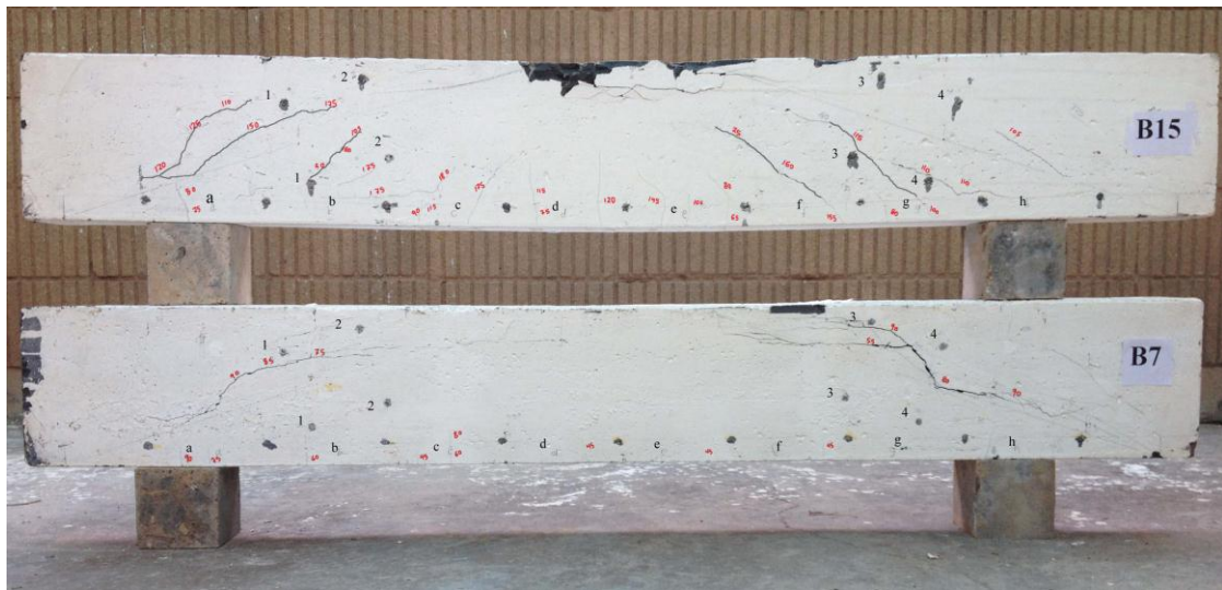
Plate 4.6 Crack Patterns of NSRPC Beams (B7,B15 with Steel Stirrups)
