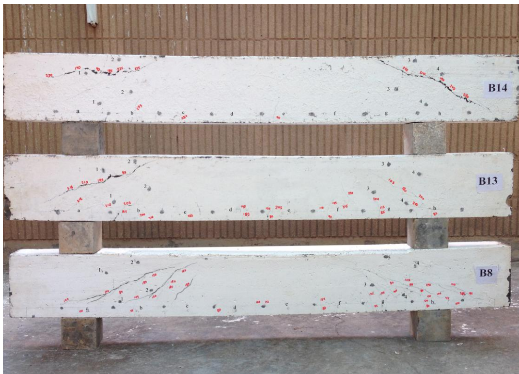
Plate 4.5B Crack Patterns of NSRPC Beams (B8,B13,B14 with Varying a/d, V_f=1\% )
