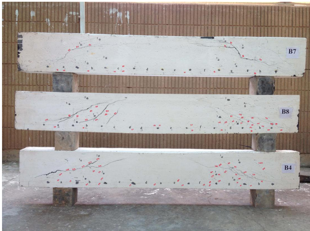
Plate 4.3 Crack Patterns of NSRPC Beams (B7,B8, B4 with Varying V_f )
