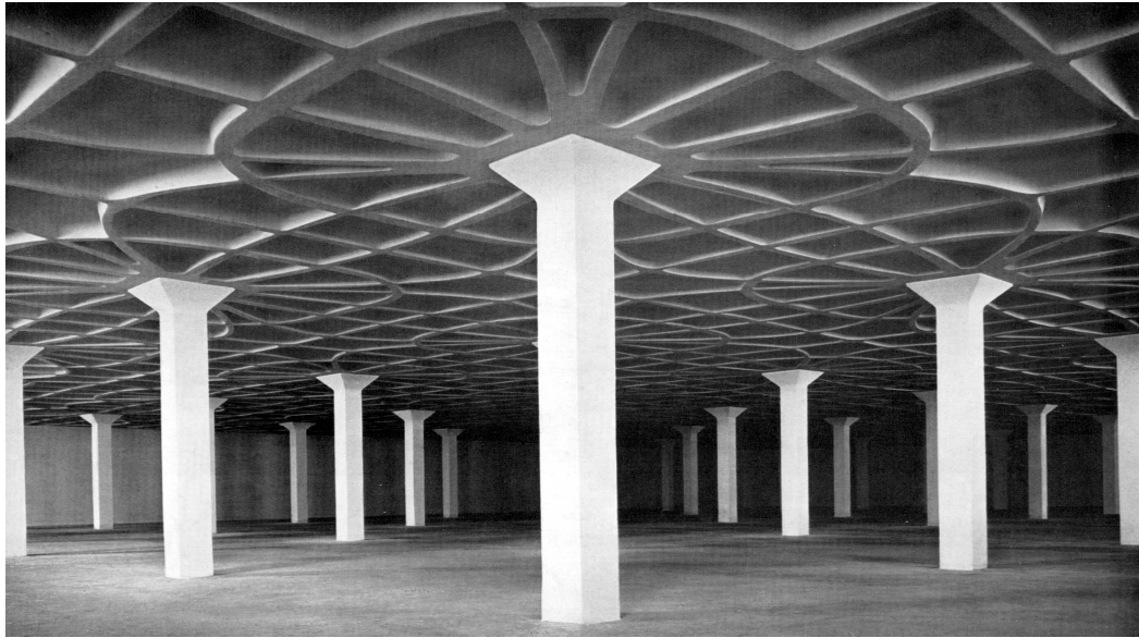
Figure 2.15 waffle slab appearance
