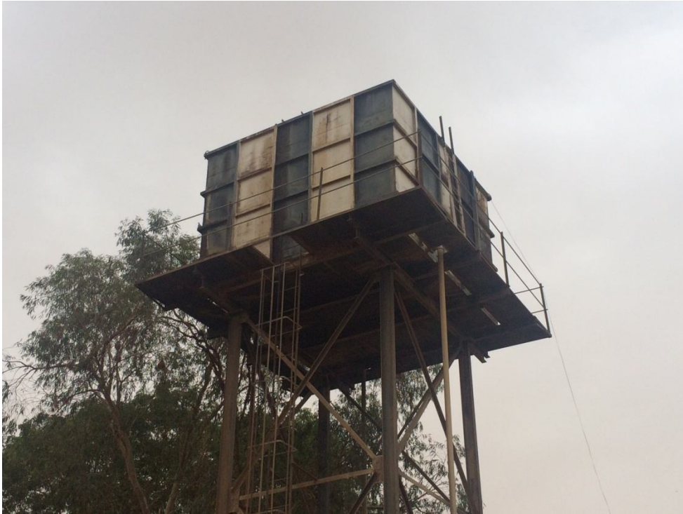
Plate (3-1) The water tank used as source of irrigation water: The dimensions 3*3*2.4 meter
