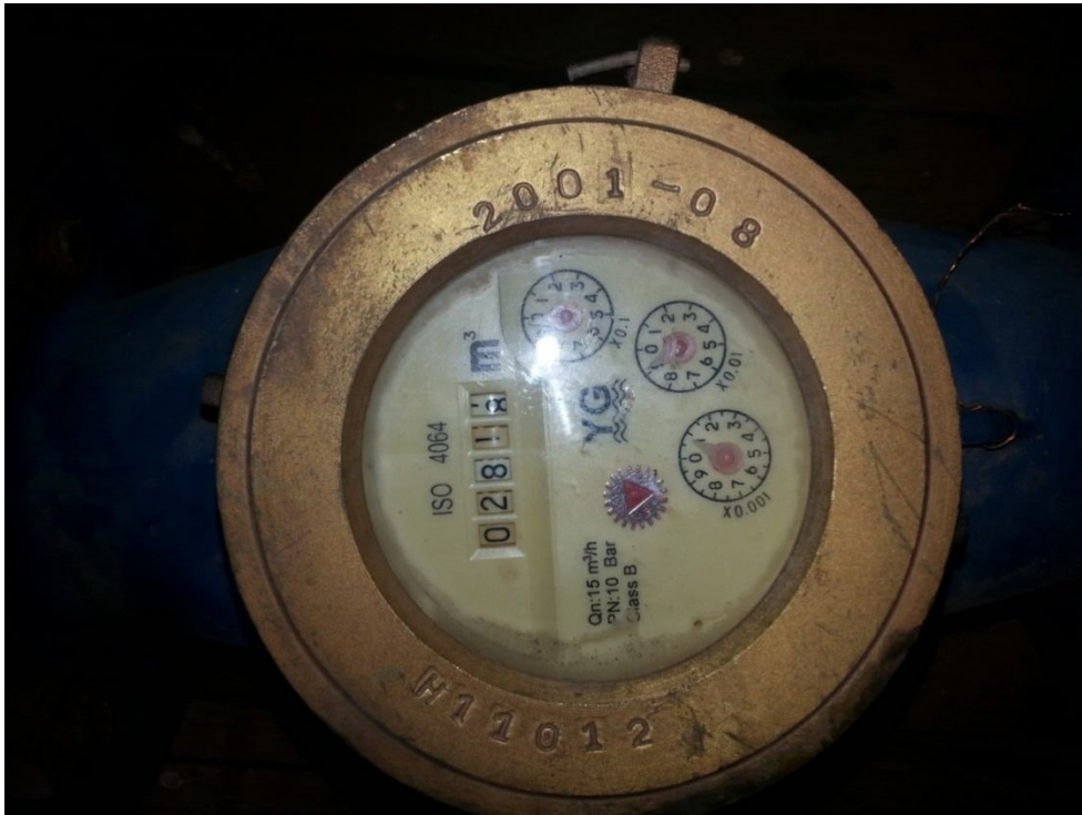
Plate (3-2) The two inch flow meter.
