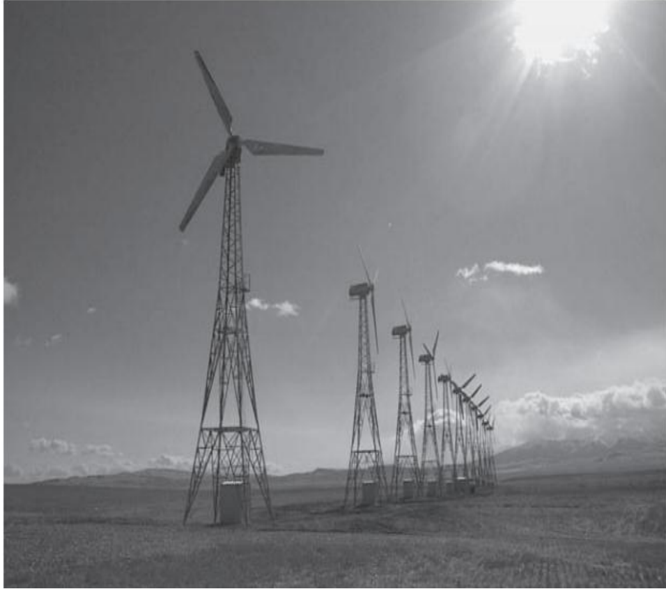
Figure (2.11) show Turbines with lattice tower.
