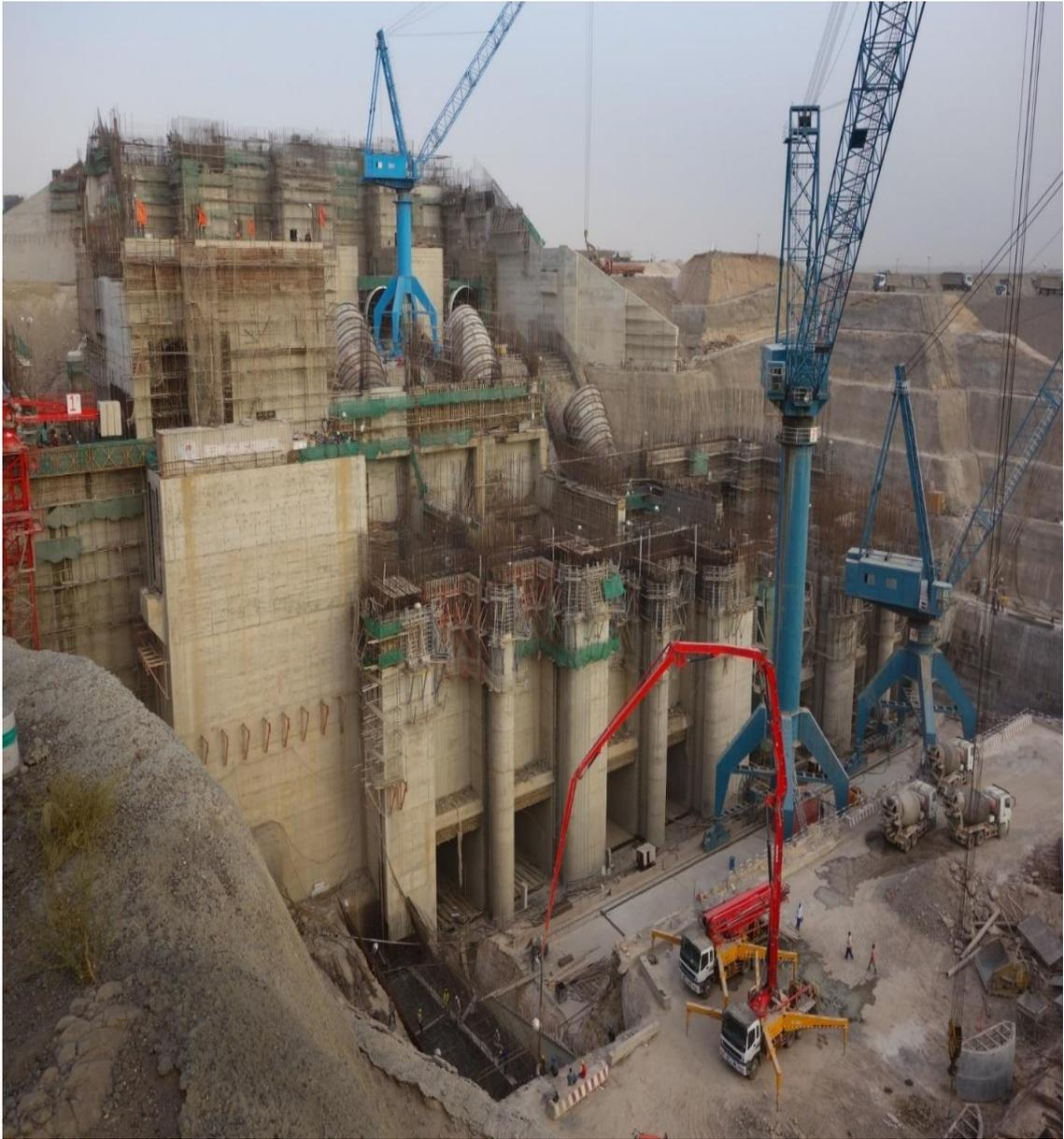
Photo B-3, DCUAP- Down Stream Power Station Concreting.
