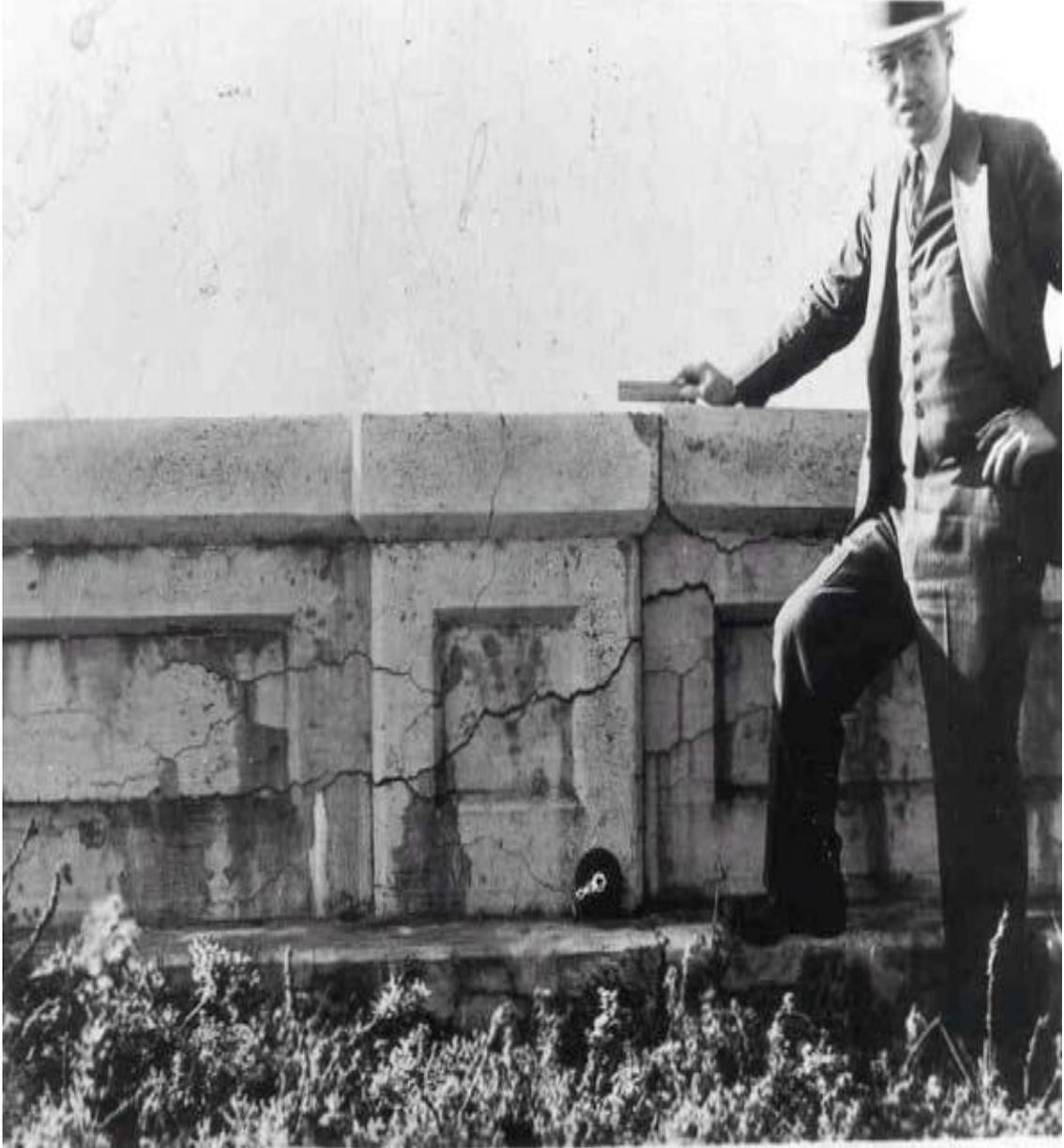
Photo B-1, Thomas Stanton of the California State Division of Highways and a Bridge Parapet Wall that is Showing Signs of Damage due to Alkali-Silica Reaction.
