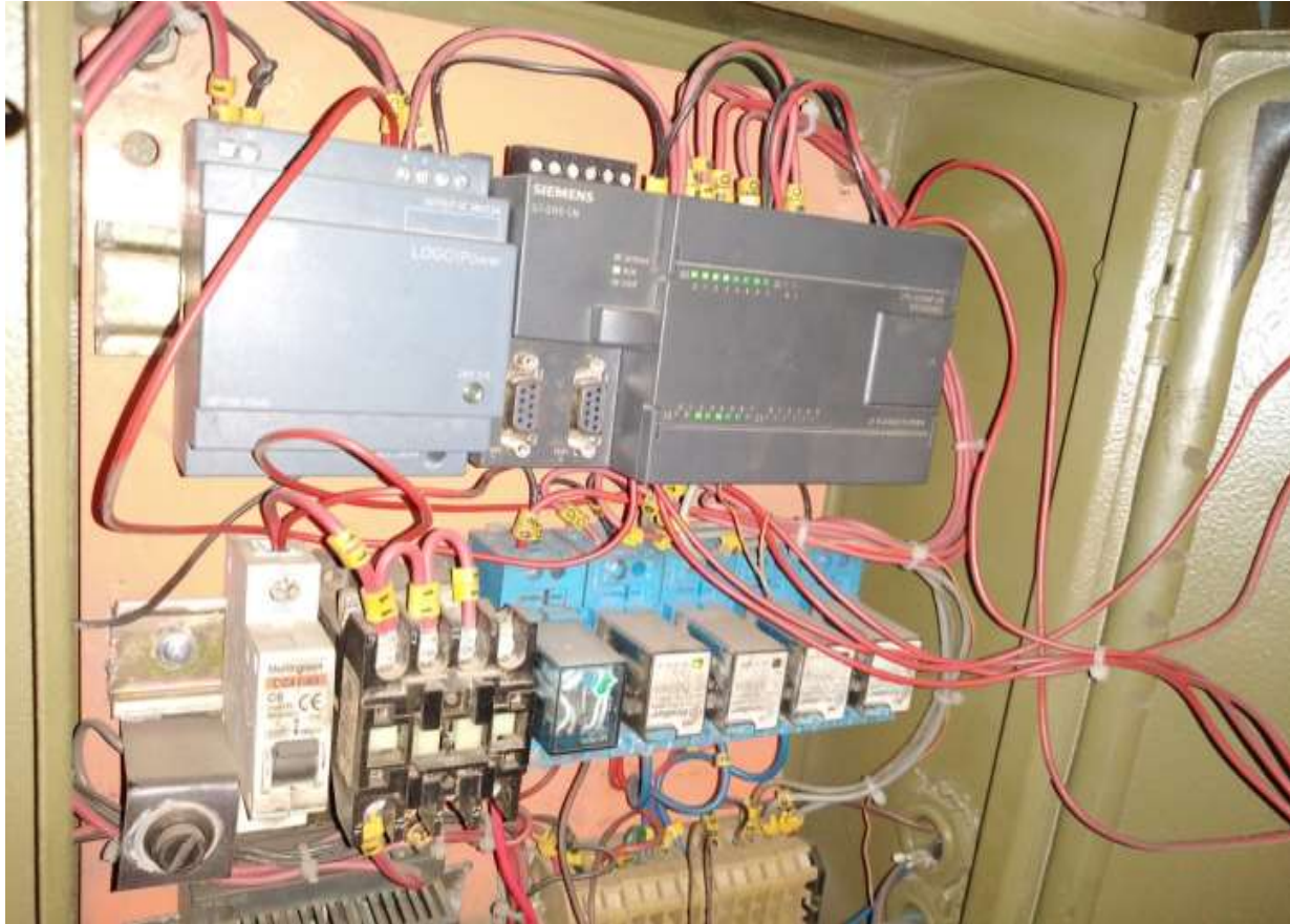
Figure 3.8: PLC Unit & Wiring
