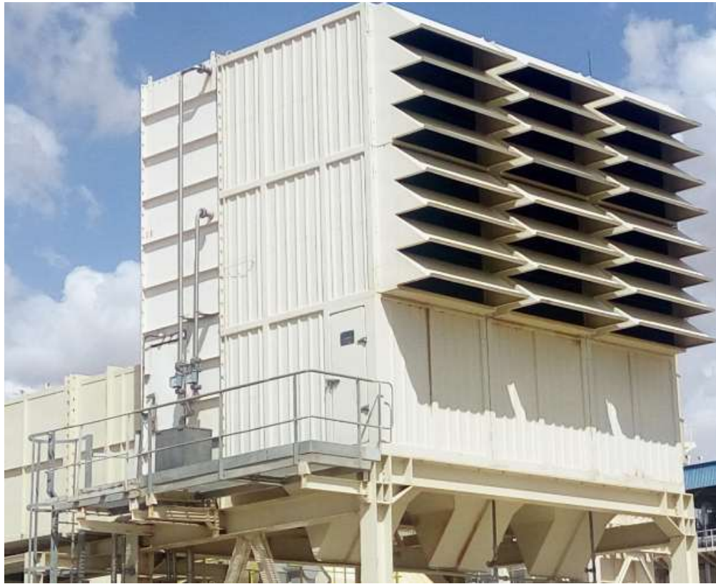
Figure (3) inlet air system
