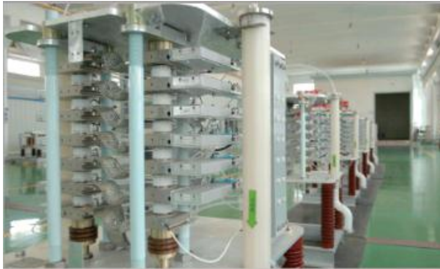
Figure A-3: Thyristor valve of SVC
