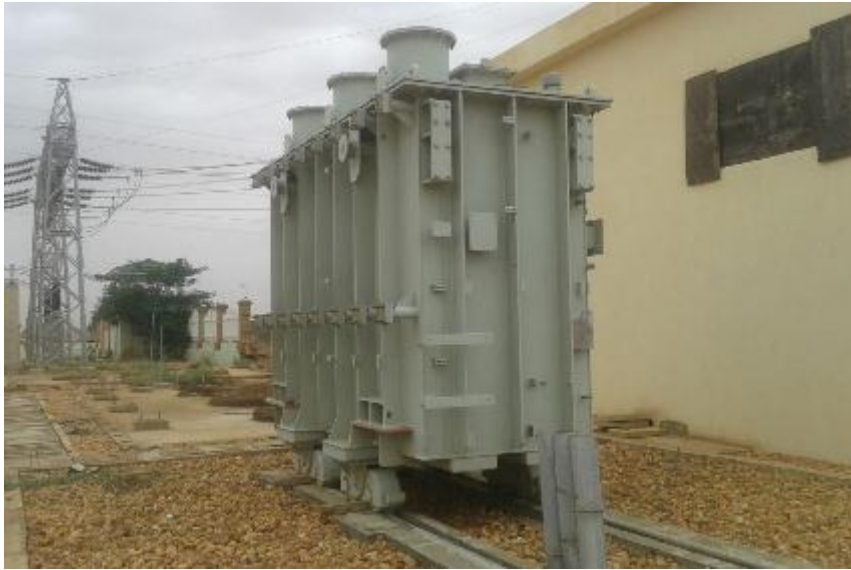
Figure A-5: Location of SVC transformer (110/33)kv
