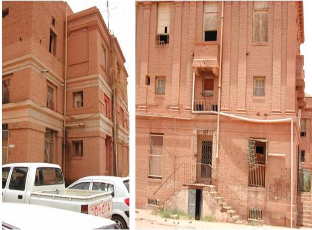
Figure 3.6(c): Scattered way for connecting sewage [16]
