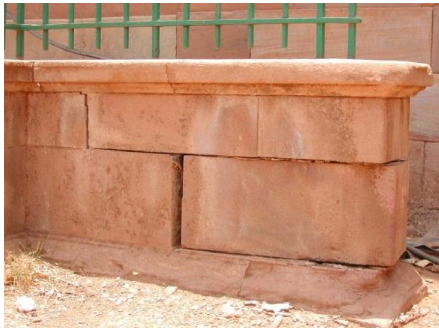
Figure 3.4(c): Loose masonry units [16]
