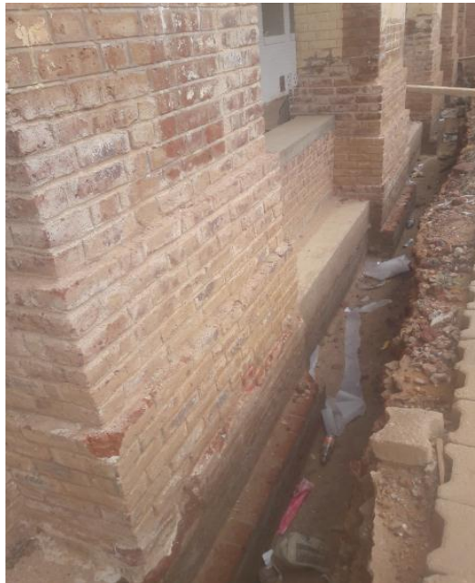
Figure 4.8: Excavate foundations for maintenance
