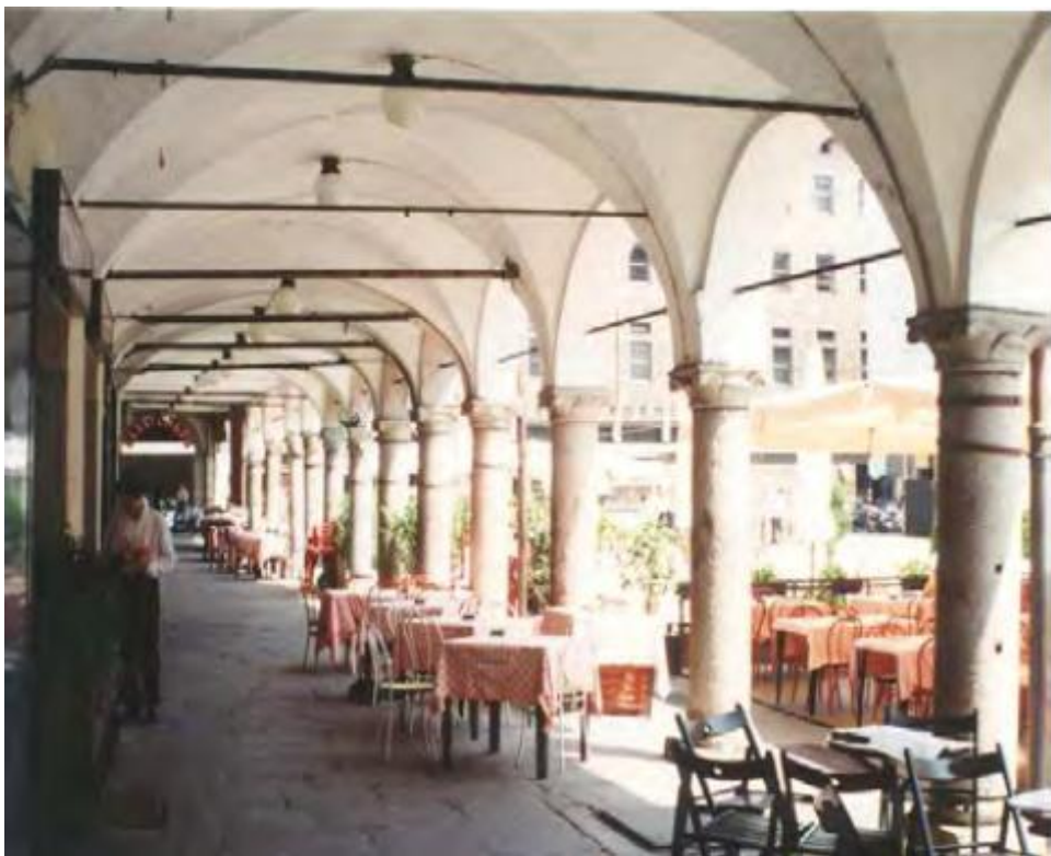
Figure 2.21: Tying of masonry vaults with tie-rods in steel
