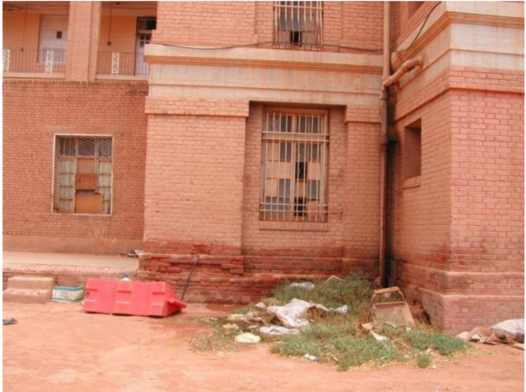
Figure 3.4(d): Damp walls [16]
