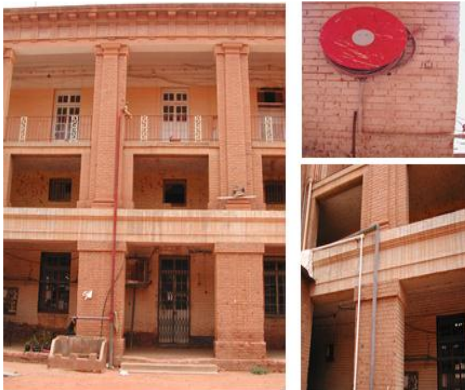
Figure 3.6(d): Scattered way for connecting firefighting [16]
