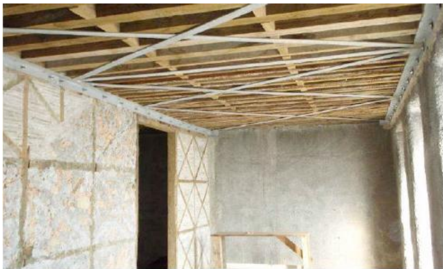
Figure 2.18: In plane stiffening with metallic diagonals and reinforcement of connection floor wall
