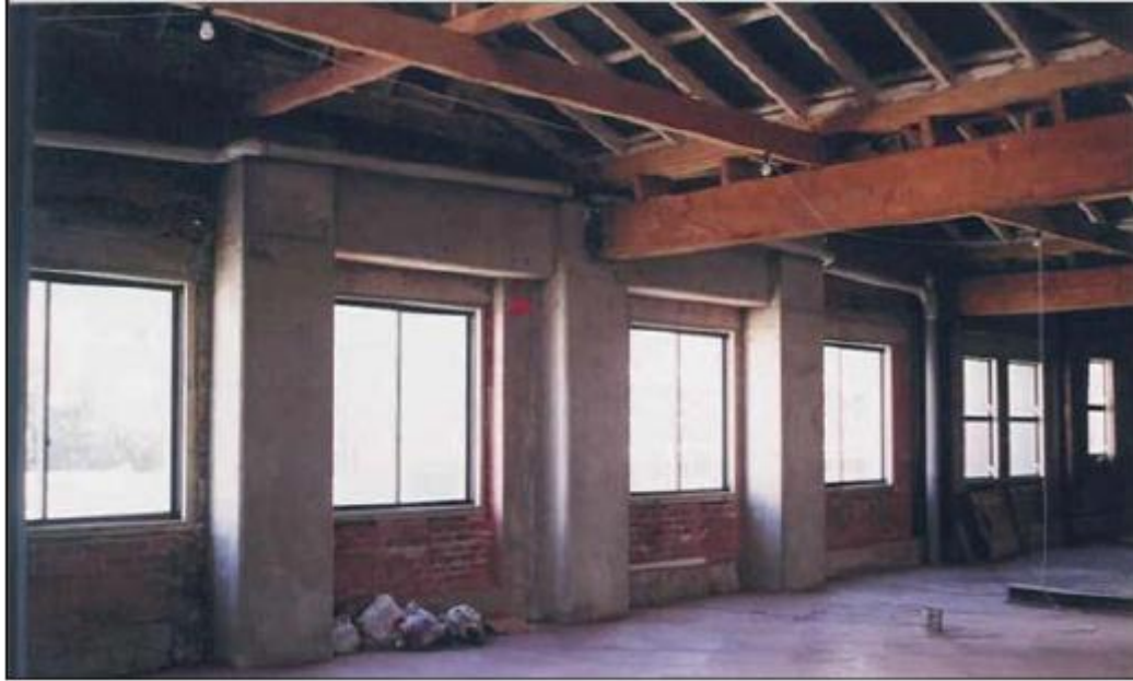
Figure 2.25: A concrete moment frame inside the façade of a large URM building in Wellington
