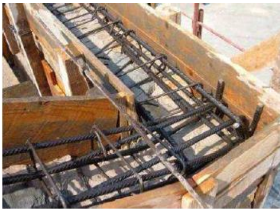
Figure 2.23: Details of the reinforcement of the ring beam (left) and view of the ring beam after filling with the concrete
