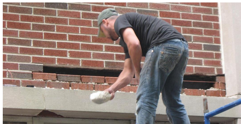
Figure 2.6 Bricks replacement
