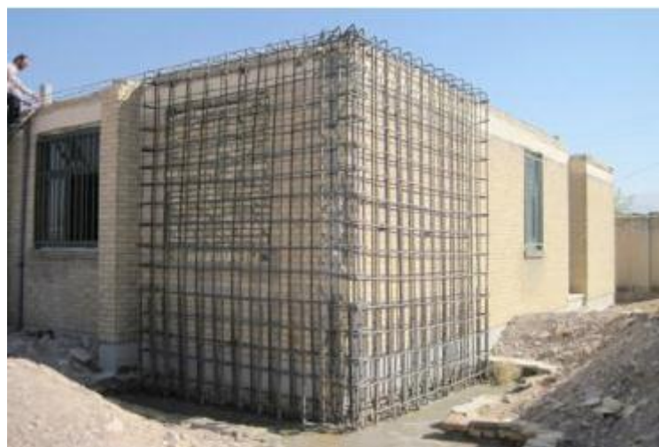
Figure 2.24: Photo of the reinforcement of two perpendicular shear walls
