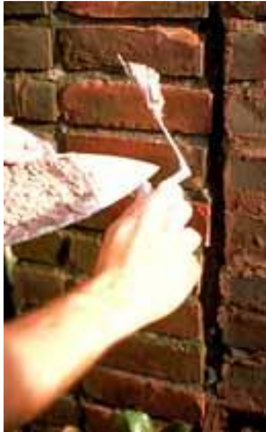
Figure 2.5: Soft mortar for repointing
