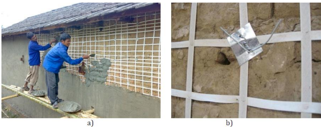
Figure 2.16: a) Implementation of PP band method of retrofitting in Kathmandu Valley b) anchorage throughout the wall
