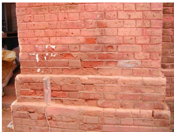
Figure 3.4(a): Disintegrating mortar [16]
