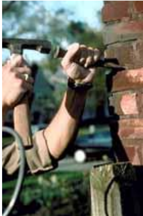
Figure 2.4: A hammer and chisel are being correctly used to prepare a joint for repointing
