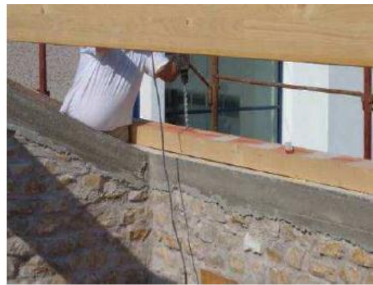
Figure 2.23: Details of the reinforcement of the ring beam (left) and view of the ring beam after filling with the concrete
