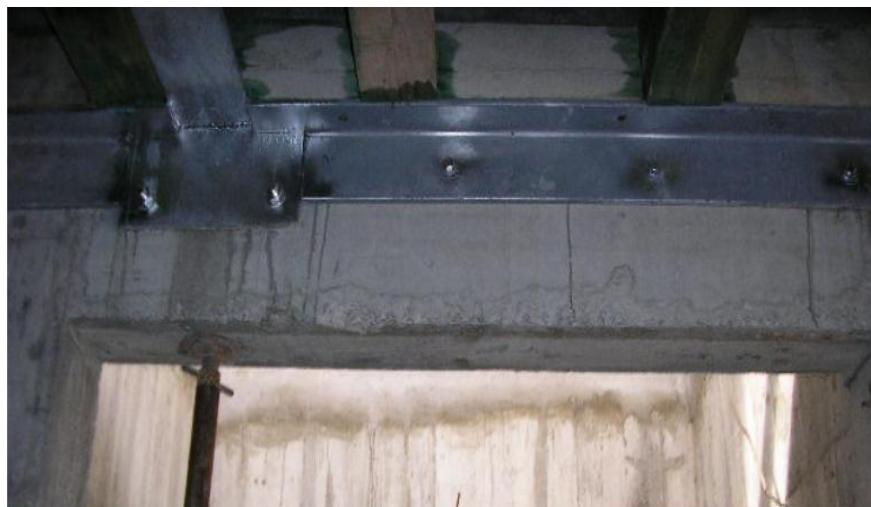
Figure 2.19: Photo of the connection with L-shaped steel plates between wooden floor and masonry wall
