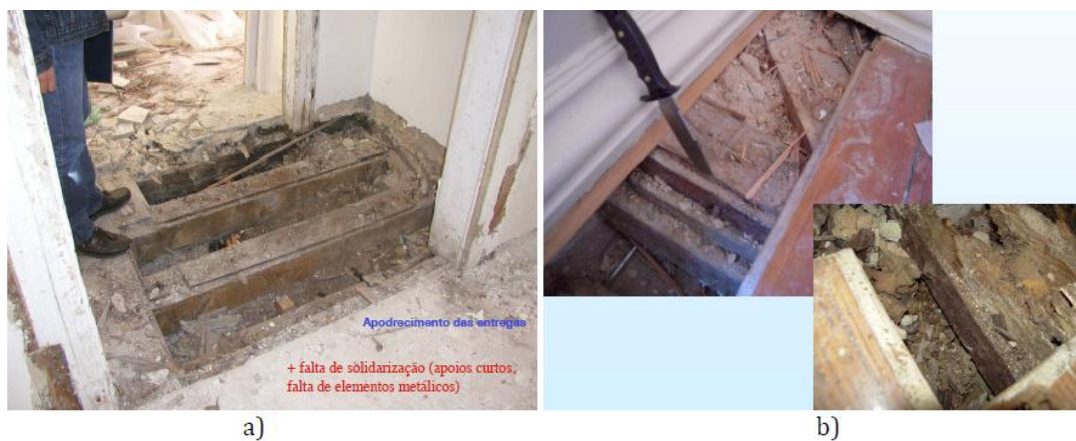
Figure 2.14: a) Rotten wood joists at the connection to the wall; b) Rotten wood elements
