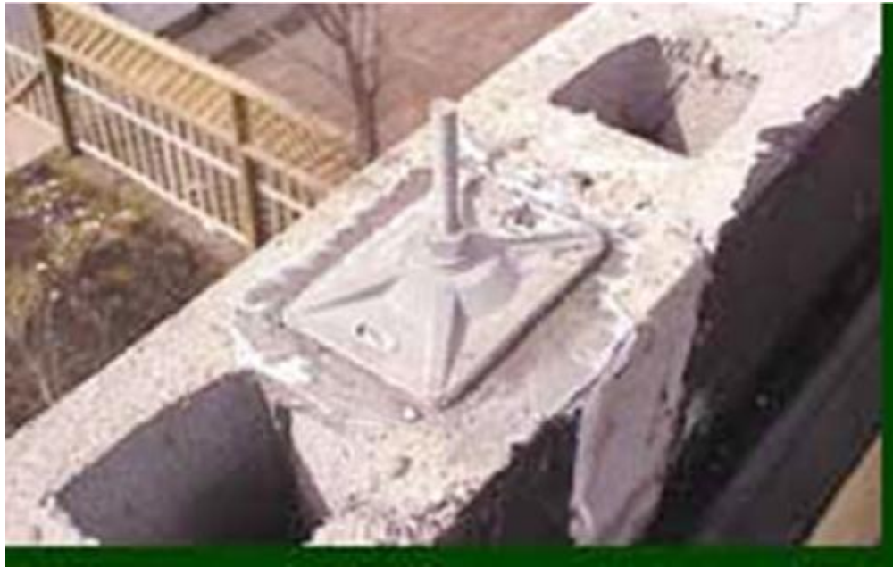
Figure 2.22: Close-up view of a post-tensioning anchorage
