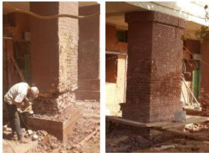
Figure 4.9: Bricks replacement in columns [15]
