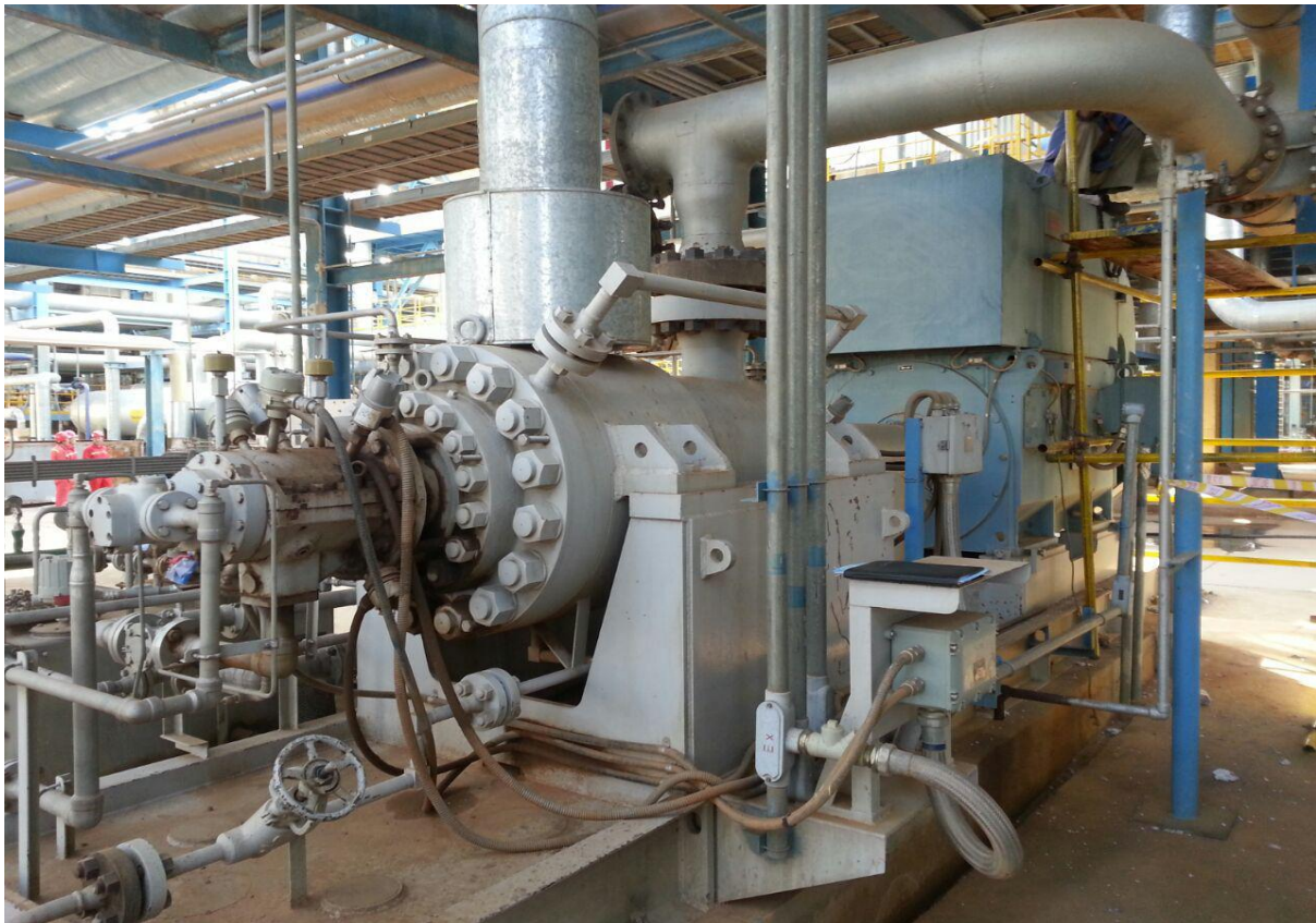
Figure (3-10) multi stage centrifugal pump
