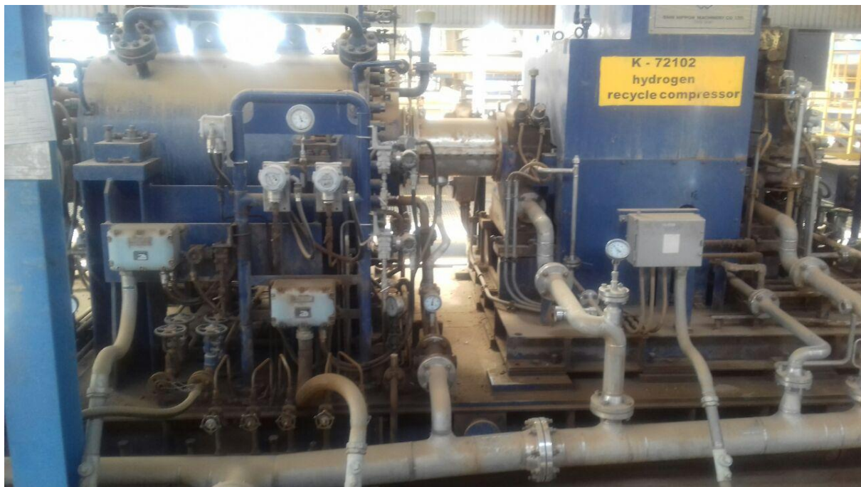
Figure (3-4) multi stage centrifugal compressor
