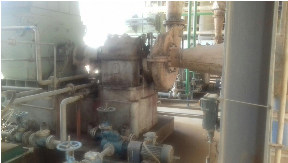
Figure (3-6) single stage centrifugal compressor
