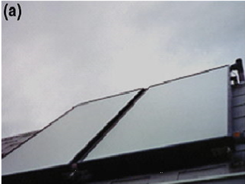
Fig (2.3 a): Shows flat plate collector
