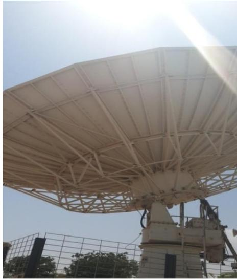
Figure 4.10: 11.2 m Antenna Hub
