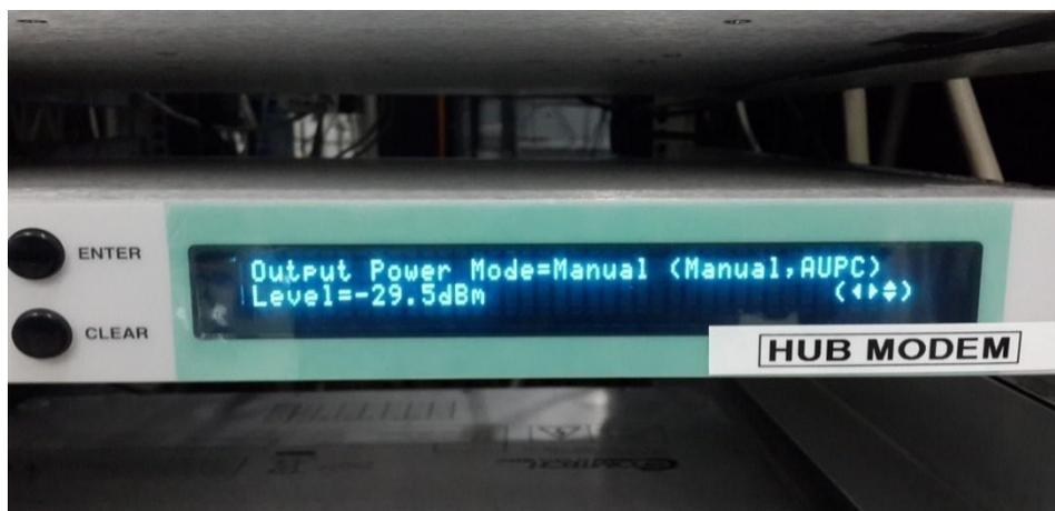
Figure 4.17a : Hub modem power adjustment
