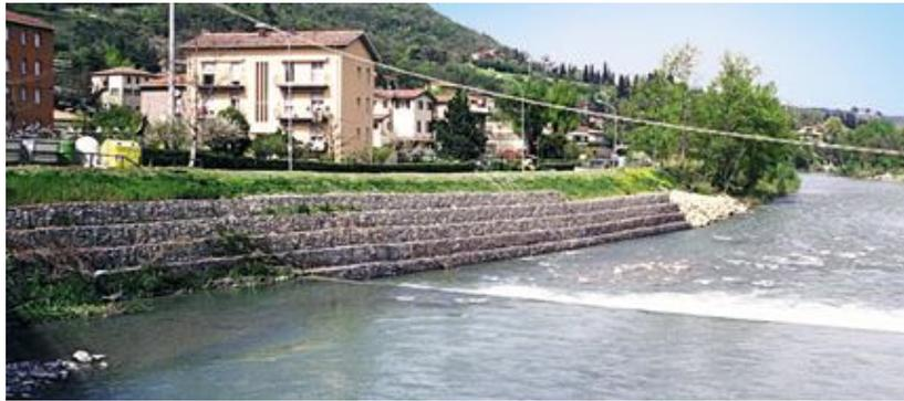
**Figure (517): Typical Guide Bank Gabion Walls**
