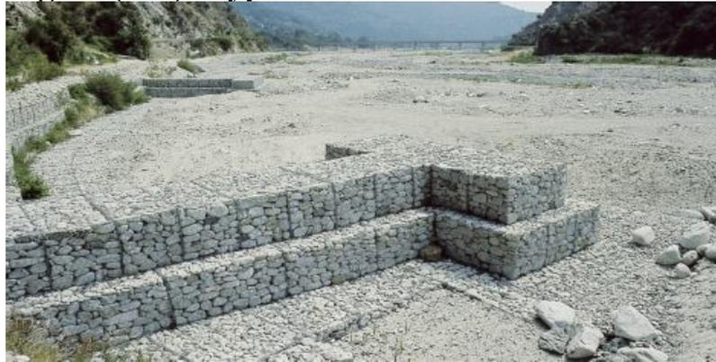
**Fig.(5.18): Typical Gabion Groins Construction**
