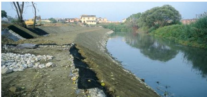
**Fig. (5.19): Guide Bank Failure**
